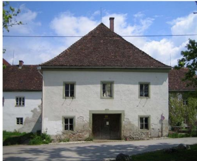
Front view of the building before renovation.
