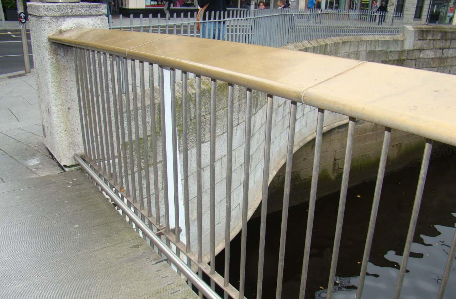
**EXAMPLE OF STAINLESS STEEL BALUSTRADE WITH A BRONZE ALUMINIUM HANDRAIL**
