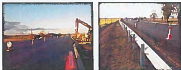
N76 Callan Road Realignment – New Road Construction
