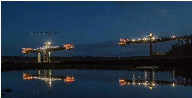
A nighttime image of the Rose Fitzgerald Kennedy Bridge under construction
