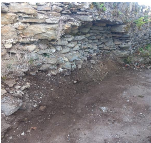
Wall Collapse at Cloghabrody
