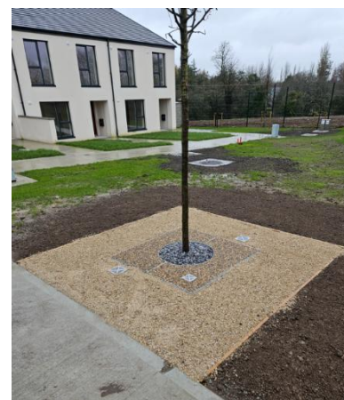
A tree pit system installed at Corkers Hill, Kilkenny
