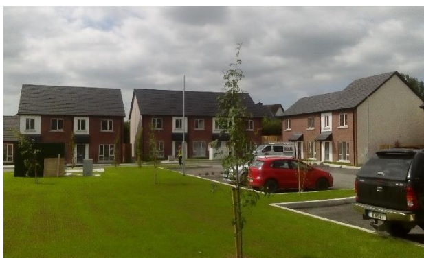
54 units Ballybough Street, Kilkenny - Respond Housing
