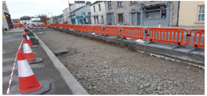
N77 Ballyragget- Works in progress on the reconstruction of failed pavement
