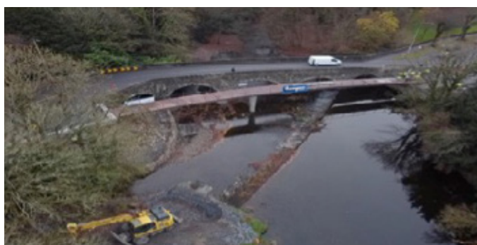
Overview with the new Castlecomer Footbridge in position (just after the bridge lift)
