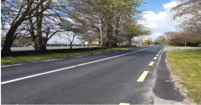
N78 Baun to Hennebrys Cross- Finished Pavement at Dunmore
