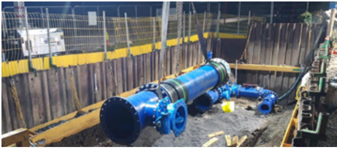
PRV installation at Radestown WTP
