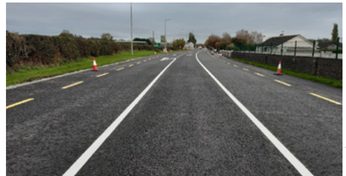
N77 Oldtown to Ballyragget – Finished Pavement
