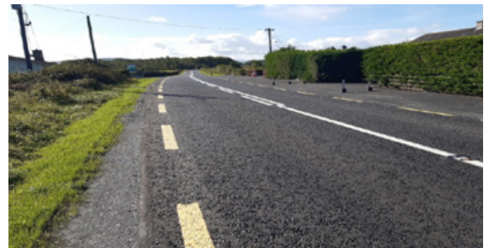
N76 Riversfield to Ahanure North – Finished Pavement
