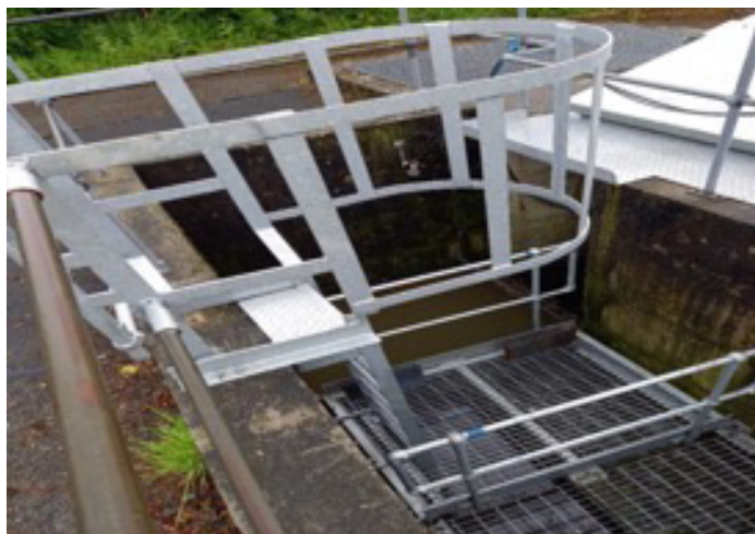
New Access Platform with Handrail support at Paulstown WWTW
