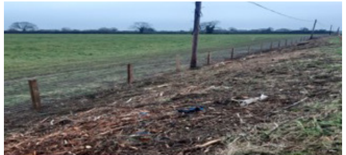
Typical Fencing Retrofit completed works on the N76
