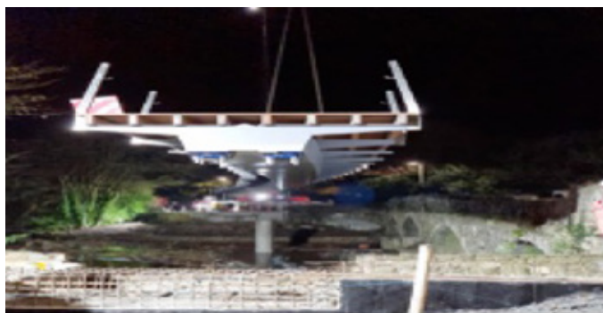
Bridge Lift in Progress around midnight on night of 23rd November
