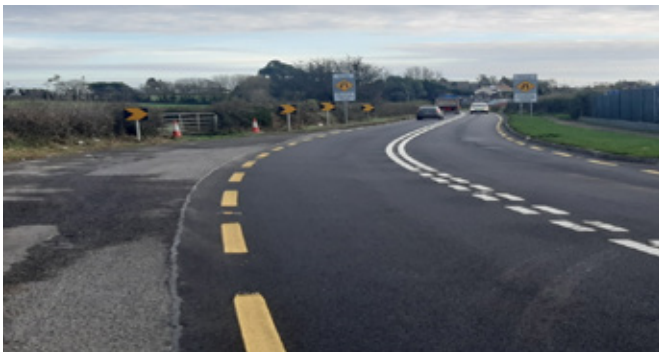
N24 West of Mooncoin. Renewed pavement, markings and signage.
