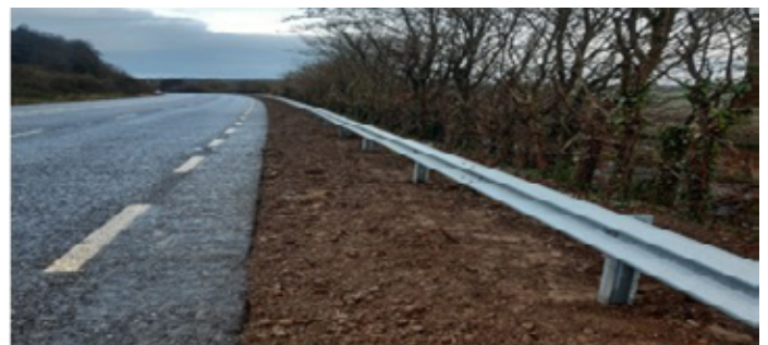
New section of VRS on the R723 (Former N25)
