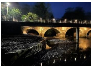
New Pedestrian Bridge, Castlecomer
