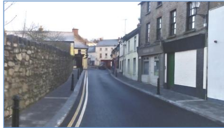
Pipe Street – After
