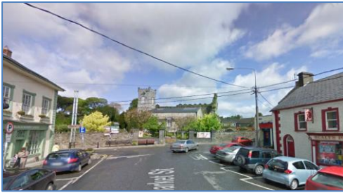
Thomastown-Market Street – Before
