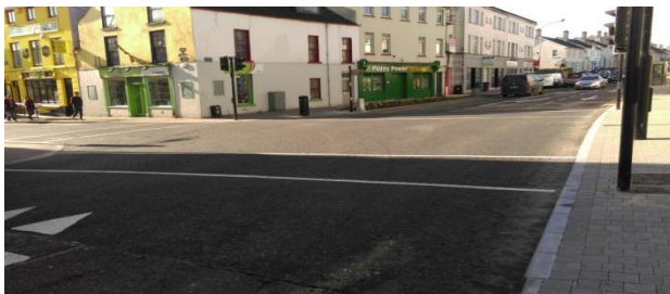
Irishtown Junction Before Works
