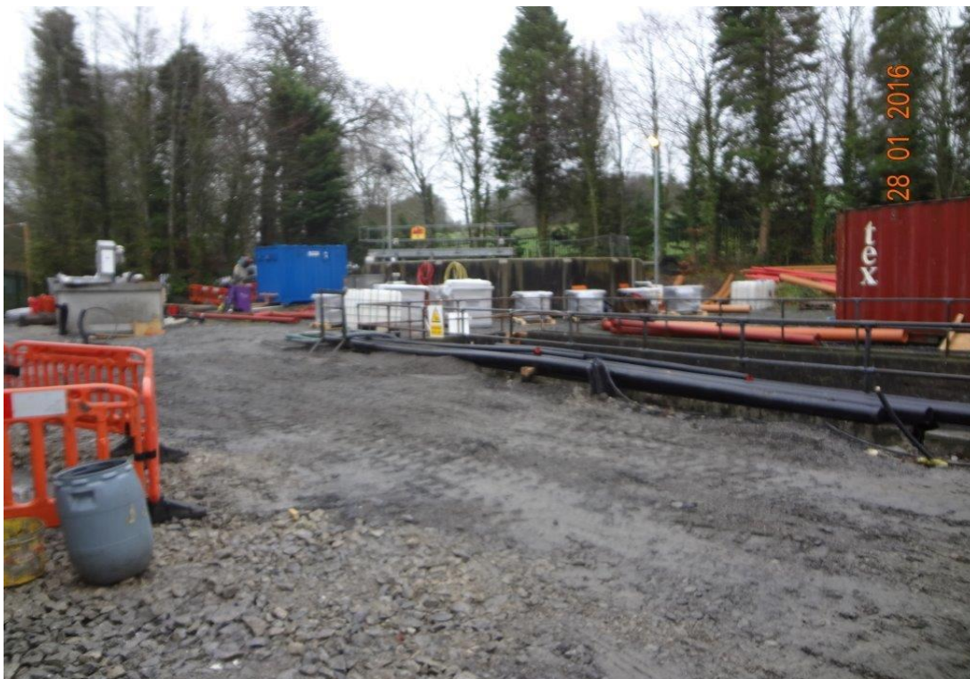
Castlecomer Wastewater Treatment Plant - Works in Progress
