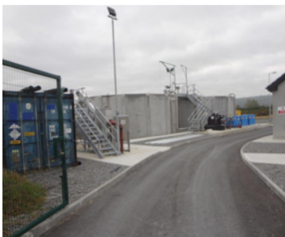
Freshford Waste Water Treatment Plant
