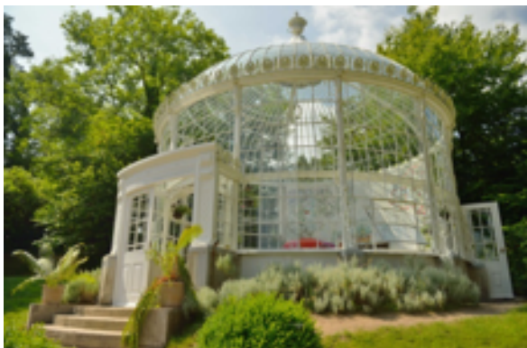
The Turner Conservatory in Woodstock which houses the tea room
