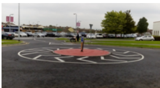
Completed works at Bohernatounish Road
