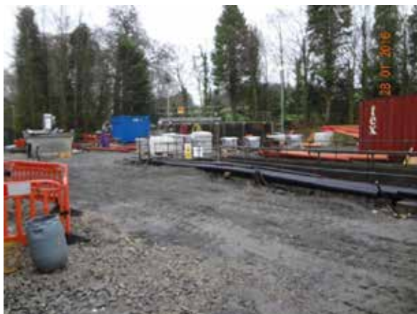
Castlecomer Wastewater Treatment Plant - Works in Progress.
