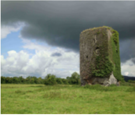
Castle Field, Sandfordscourt
