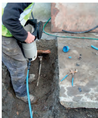
Water conservation main rehabilitation works at John's Quay in December 2013
