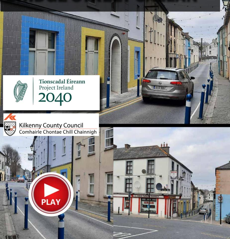
Funding was secured towards improvement to public realm space on Bridge Street Callan to accommodate cycle tracks and shared surfaces for walking, age-friendly and improving social distancing. Bollards, road markings, signage and realignment works at junction to accommodate same were all put in place.
