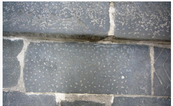
Typical 18 th Century worked stone paving and step detailing, disturbed and reset.
