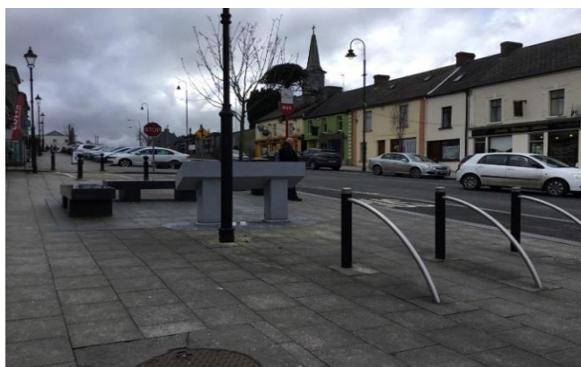
Figure 14. Bicycle parking facilities on Green Street
