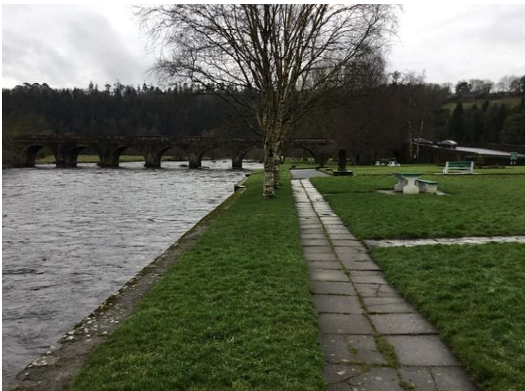
Figure 45. Riverside Park / The Green and Ten Arch Bridge.
