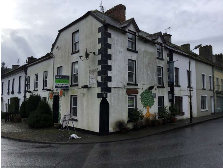
Figure 32. Prominent Vacant building overlooking Riverside Garden
