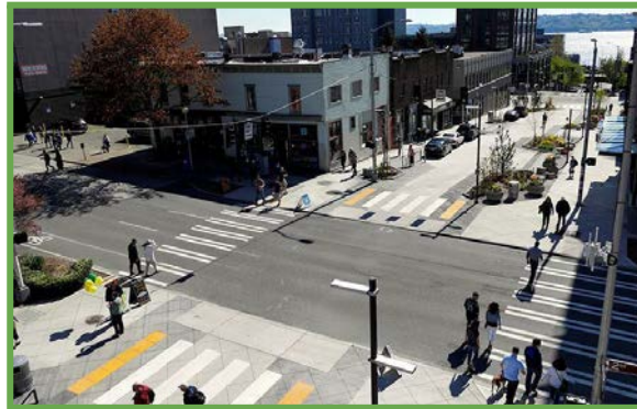
Bell Street Park, Seattle: This design is user friendly for all, especially visual impaired by eliminating curbs, creating open clear space with tactical signs. The Narrow lanes and parking help slow traffic.
