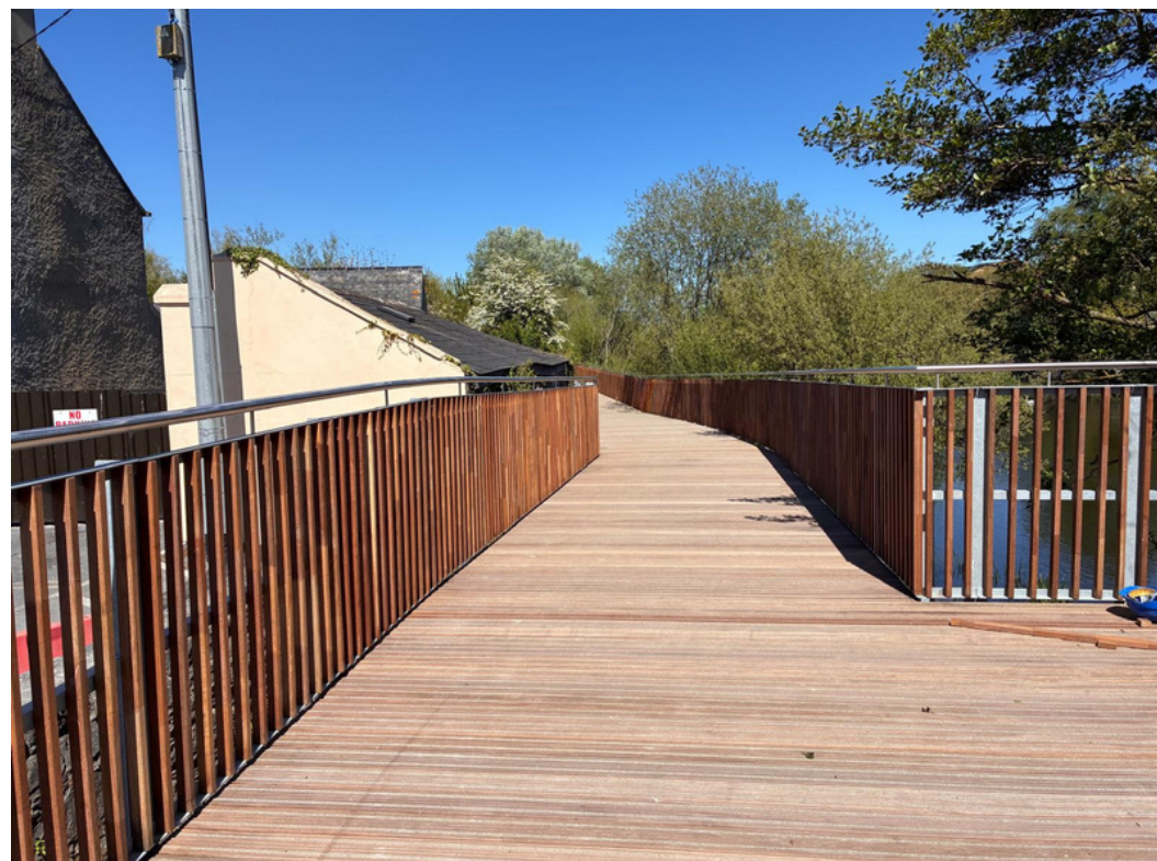
Boardwalk at Greensbridge
