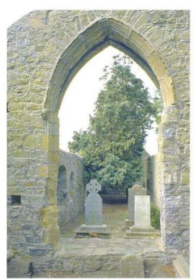
Above The use of cement mortar and ribbon pointing, as shown here, is inappropriate in the conservation of medieval buildings.
