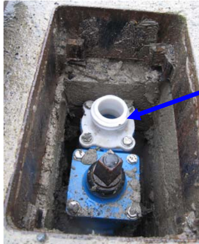
Figure 4.0 – Plastic/nylon outlets on hydrants
