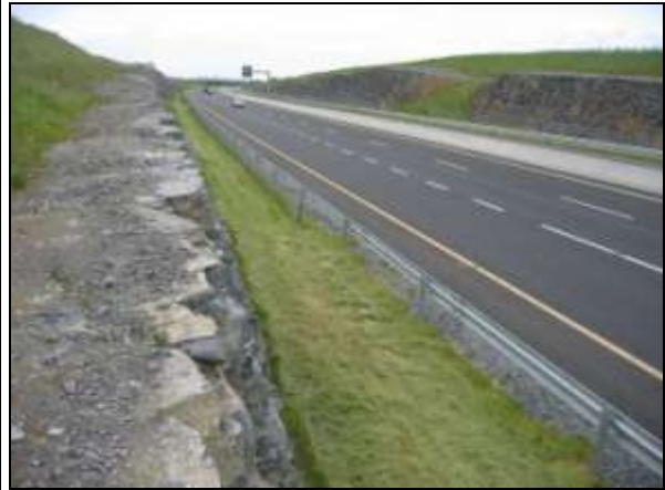
General view looking north.
