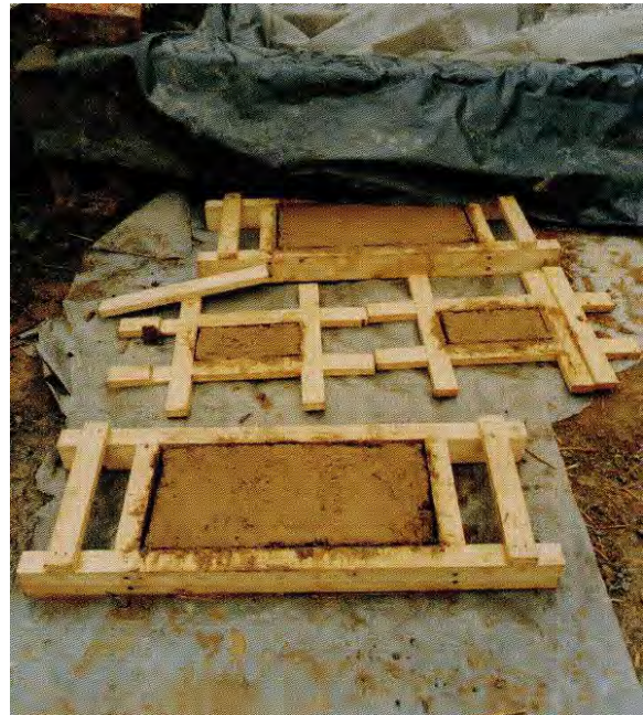
Mud bricks, formed in wooden moulds, were used to repair decayed parts of the mud walling (Heritage Council)
