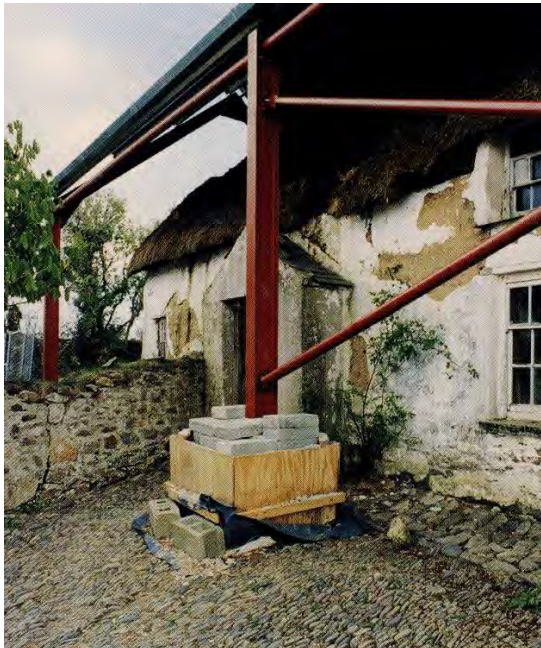
A temporary protective shed was erected over the building to facilitate conservation works (Heritage Council)
