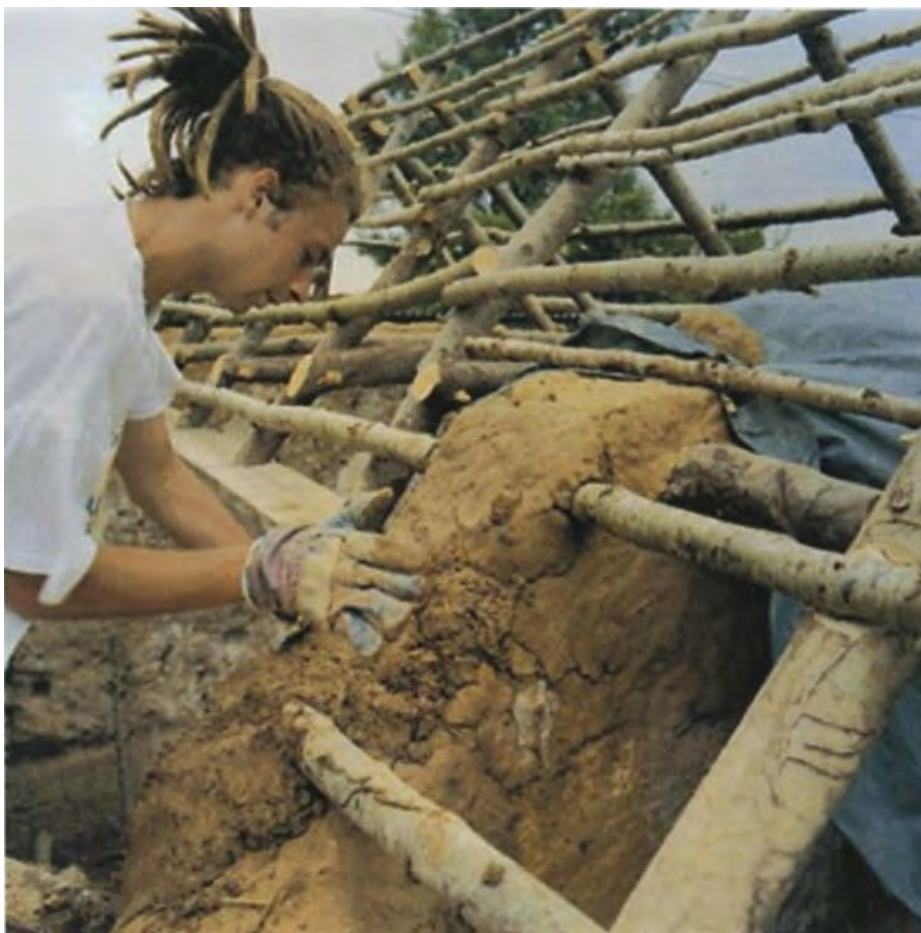
Repairing mud walling, Mayglass, Co. Wexford (UCD)
