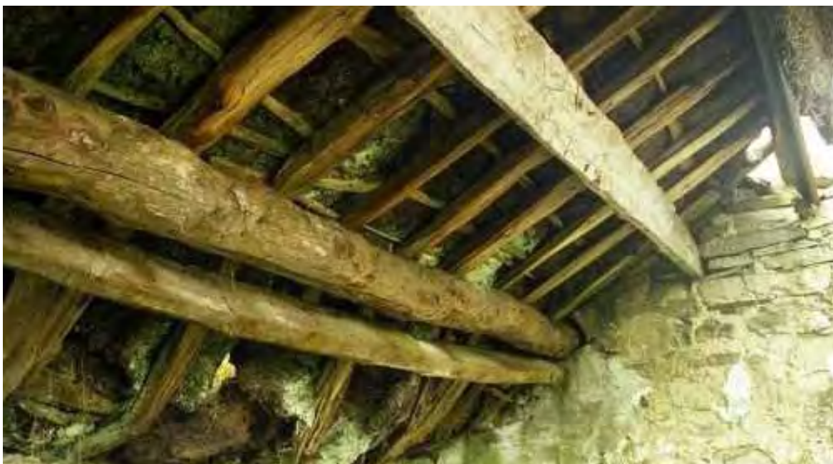
Historic thatched purlin roof structure, near Mullaghmore, Co. Sligo (Barry O'Reilly)
