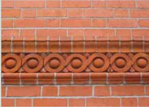
A example of the decorative use of moulded brickwork and terracotta in a stringcourse
