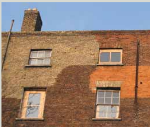
The gutters behind parapet walls are difficult to access and therefore are often poorly maintained. Many parapet walls show evidence of having been reconstructed over the lifetime of the building. This illustration shows the use of inappropriate replacement bricks in the repair of the wall
