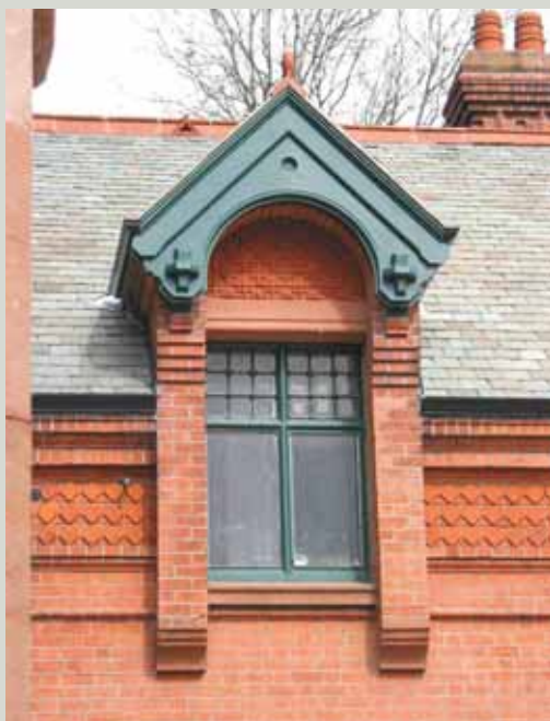
The Red Stables, St Anne's Park, Raheny, Dublin, built in 1886 of machine-made brick from the Portmarnock Brickworks
