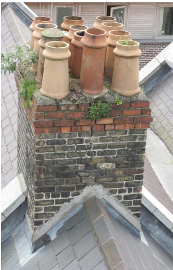
Figure 35: Traditional chimney stack requiring repair and maintenance
