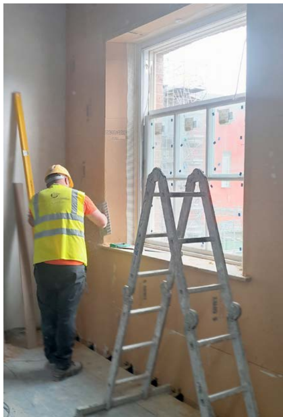
Figure 51: Woodfibre insulation board being prepared prior to application of finish coat
