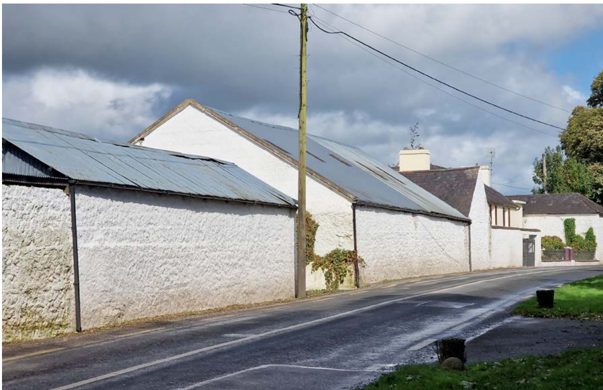
Figure 12: Limewash on traditional farm buildings
