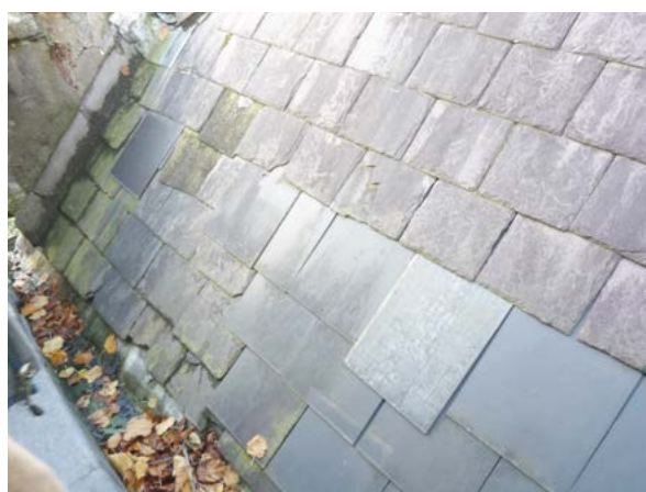
Figures 19, 20, 21: Examples of where asbestos can be found in a traditional building – panels of corrugated roof sheeting, floor tiles and roof tiles
