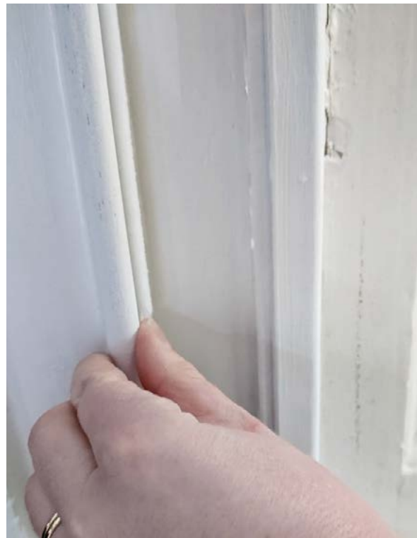
Figure 49: Discreet draught-proofing brush on a historic window
