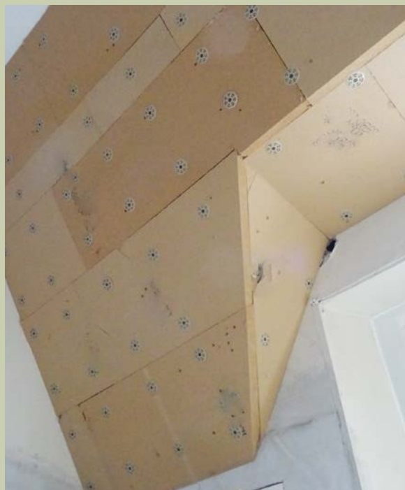
Figure 34: Wood-fibre insulation board fixed to the internal face of rafters. Thermal modelling may be required to ensure the minimum surface temperature is achieved in accordance with TGD L, Appendix D
