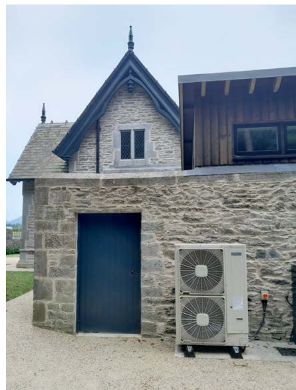
Figure 63: Air source heat pump
