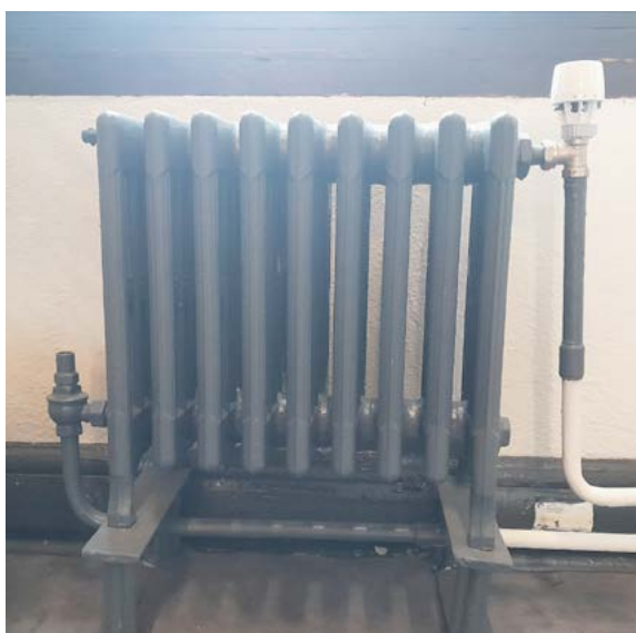
Figure 23: Cast-iron radiator with a thermostatic control
