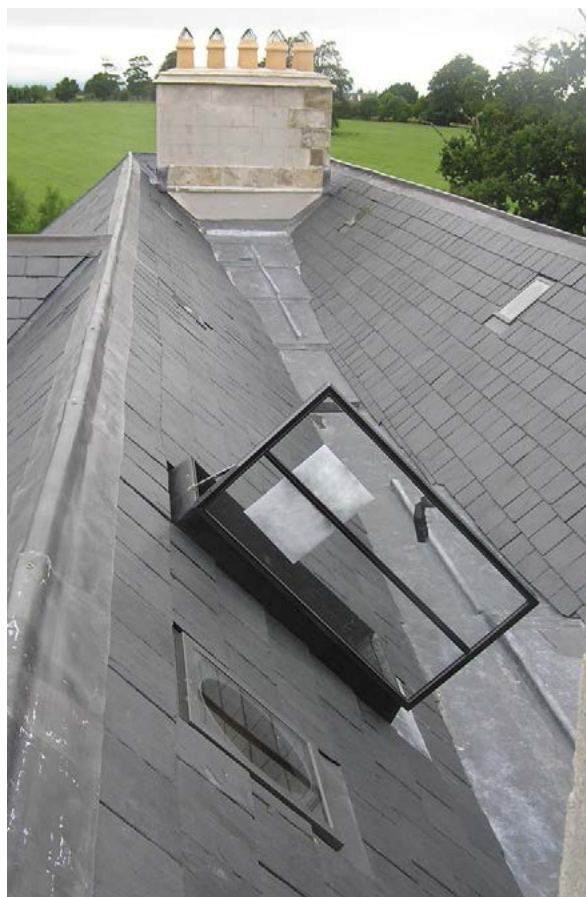
Figure 36: This modern double-glazed skylight allows access to a concealed valley gutter for maintenance inspections and cannot be seen from ground level (Image from Advice Series: Roofs , 2010)
