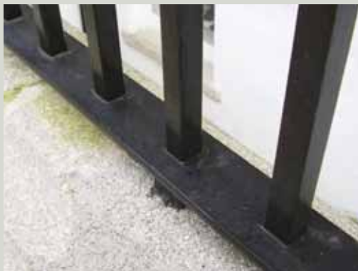
Replacement bars should pierce through the rail rather than be welded to it (as shown above)
