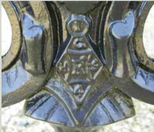
Registration marks will give the year in which a particular design was registered
