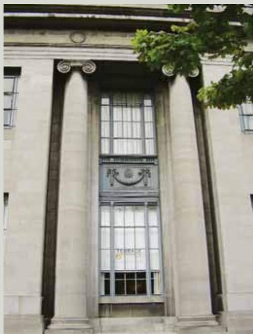
The National Concert Hall, Earlsfort Terrace, Dublin. Cast iron windows and spandrel panels became increasingly widespread from the start of the twentieth century. This example was supplied by the Scottish firm Walter Macfarlane & Co. Ltd in 1914
