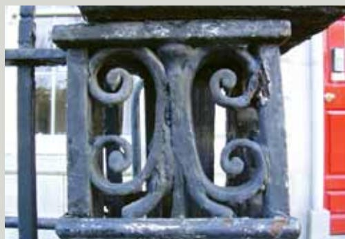
Posts from two different properties on Parnell Square, Dublin. While appearing to be severely corroded, much of the original ironwork in the lower example may remain intact beneath layers of paint and corrosion
