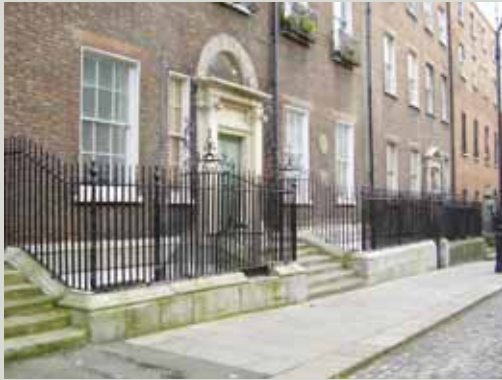
Early eighteenth-century wrought iron railings, Henrietta Street, Dublin. The large-scale development of squares and terraces from the 1700s onwards fuelled a rising demand for iron railings
