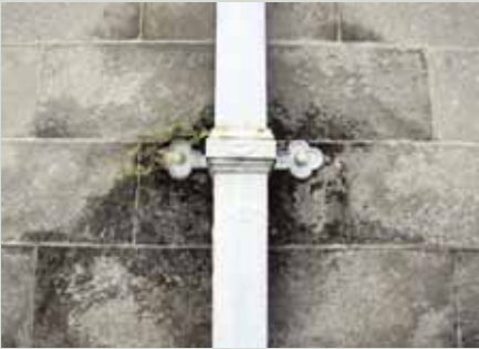
The staining of the stone wall behind this downpipe joint suggests there is a blockage inside the pipe. If the water trapped inside freezes in cold weather, it may burst the pipe
