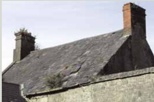
The roof provides the first line of defence for the interior of a building against the weather and it is essential it is well-maintained and kept in good repair
