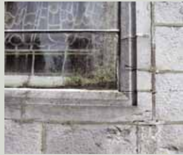
Poor ventilation of the space between a stained glass window and new storm glazing has created so much condensation that plants can now grow which will damage the stained glass panel
