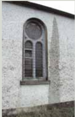
Inspecting a building during, or immediately after, a downpour can be a useful way to discover defects in rainwater goods. In this case, it is easy to spot the location of a leak in the gutter
