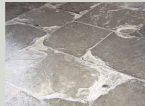
Stone flags in basements were often laid directly on the earth below. It is essential that their surfaces are not sealed or the joints between flags filled with cement as this will trap moisture in the stone and cause decay
