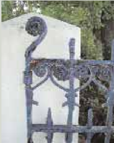
Wrought ironwork was traditionally made in a forge by a blacksmith hammering the material into the required shapes. It is essential to keep the paint covering intact on both wrought and cast iron to prevent corrosion.
