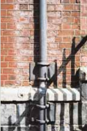
A white bloom of salts deposited on the surface of a wall, known as efflorescence, usually indicates saturation of the wall. In this case, the problem is almost certainly associated with the rainwater downpipe and needs immediate action to investigate the cause of the problem and to solve it
