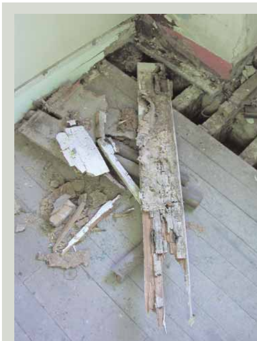
Timber which has suffered dry rot attack has a distinctive cuboidal pattern of cracking. Only timber which has decayed to the extent that it can no longer do its job should be removed in the course of treatment
