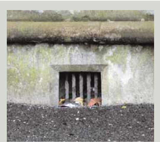
Installing hard paved surfaces around the base of a building can cause damp problems both inside and out. Here the new tarmacadamed surface is higher than the original ground level, is partially blocking an underfloor vent and making it more likely that water will flow into the building through the vent hole.
