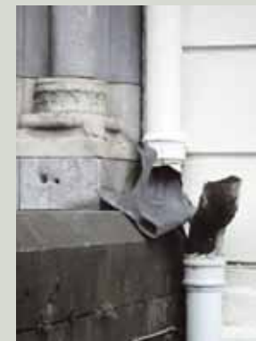
This poor quality, short-term repair of a broken downpipe, using a piece of lead to transfer rainwater from one part of the downpipe to the other, has already failed and will cause serious damp problems if not put right soon
