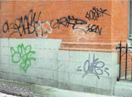
Remove graffiti as soon as possible. Not only does it disfigure the building and encourage further attack, but many paints become more difficult to remove the longer they are allowed to dry and harden
