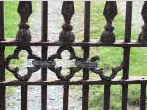
Missing pieces of decorative ironwork can be replaced with replicas cast from the original pieces
