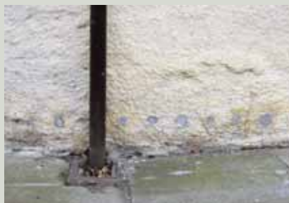
The drill holes associated with injecting a chemical DPC can be unsightly. A more effective method of dealing with the damp problem in this case would have been to reduce the level of the impermeable paving around the building and ensure that rainwater drains away from the base of the wall
