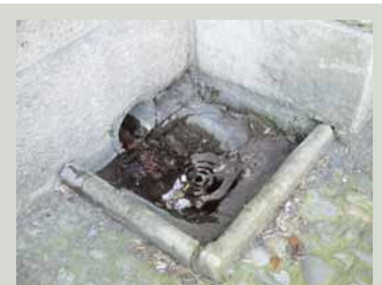
All gullies require inspection on a regular basis to ensure that litter or plant growth is not blocking the free flow of water
