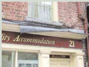
Poorly-fixed flashings may become detached and allow rainwater to soak into the building. They should be refixed or replaced as soon as possible
