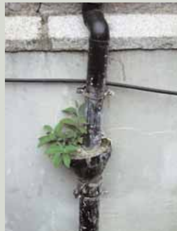
This hopper became blocked with debris during a construction project and was not cleared after the works finished. It will cause serious saturation of the wall behind if the situation is not remedied
