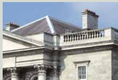
Where a building has a complex roof and other high level features that need regular maintenance and repair, providing a permanent means of safe access should be considered
