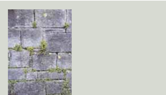
Although the plants which have taken root between the stones of this boundary wall may be visually attractive, they are a clear sign that the mortar has decayed over a widespread area, water is lodging within the wall and action is needed
