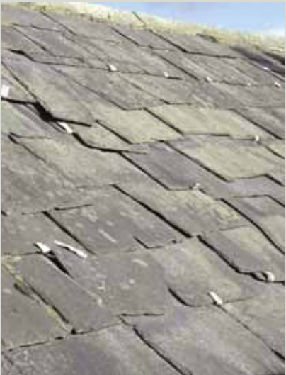
A number of tingles have been used in previous repairs of this roof but the slipping of slates continues, indicating a widespread failure of fixings. As a rule of thumb, where a third or more of slates have slipped the entire roof will require to be stripped and re-fixed, reusing the existing slates where possible
