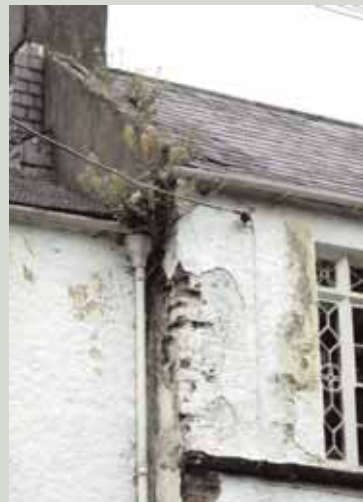
Damp problems in ground floor or basement rooms may not be caused by rising damp but by rainwater from broken gutters above saturating the wall and the ground beneath
