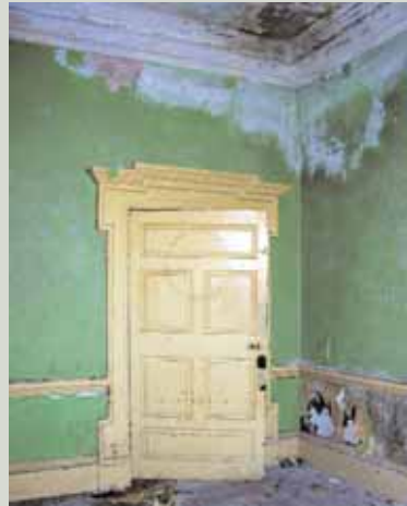
Neglect and lack of roof maintenance over a number of years have allowed water into the interior of this fine building. Redecoration will be pointless until the building is watertight again and the water already in the fabric has been given time to dry out
