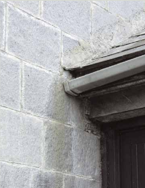
The end of this replacement gutter has not been properly fixed and has begun to sag with the weight of water trapped in it. Already the wall has been stained and there may be further damage if the saturation continues
