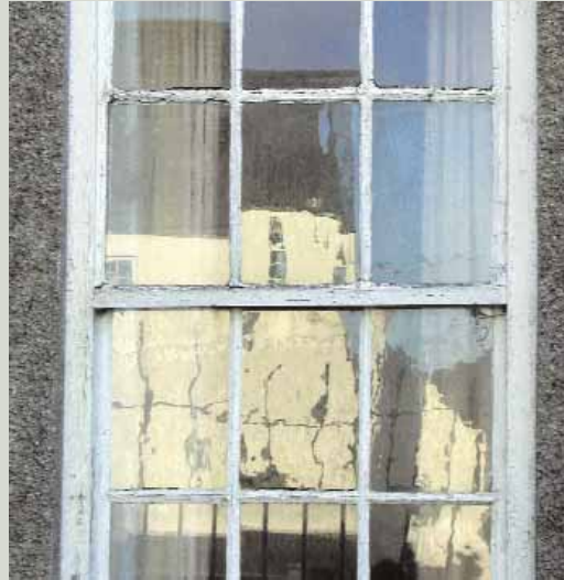
Flaking paint must be sanded or rubbed down to a sound surface before repainting. Where there are panes of historic handmade glass, care will be needed to avoid damaging them in the process
