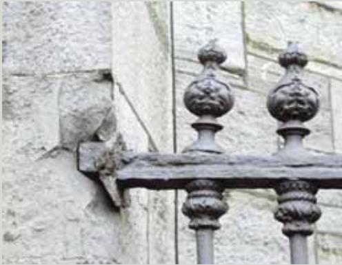
Corroding iron will expand up to ten times its volume as it rusts. Where iron that is fixed into stonework rusts, this expansion can literally blow the stone apart shattering it into pieces and exposing the ironwork to further corrosion
