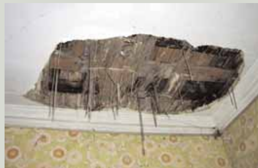
Plaster ceilings are vulnerable to the failure of their backing materials. In this unusual example, bunches of reeds, rather than timber laths, were used as a base for the plaster finish. The reeds have failed due to flooding caused by a leaking roof above and part of the ceiling has collapsed
