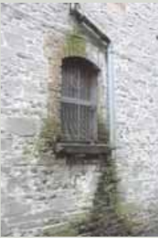
Leaking joints and missing sections of downpipe are relatively cheap and easy to fix if attended to promptly. When defects are not remedied, they lead to serious problems which are expensive to repair and involve the loss and disruption of parts of the building fabric
