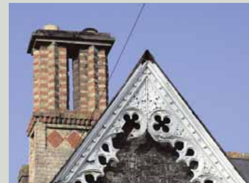
All external joinery, not just windows and doors, requires regular repainting. There may be other external timber elements that need attention including the bargeboards that trim the gable ends of a roof
