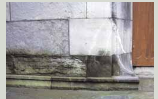
Damage attributed to rising damp may have another cause. Rainwater splashing off hard paving can soak the base of a wall, encouraging mould growth on the wet stone
