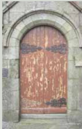
Traditionally, most external joinery was painted not just for decoration but as an essential part of its weather protection. The paintwork requires regular and frequent renewal
