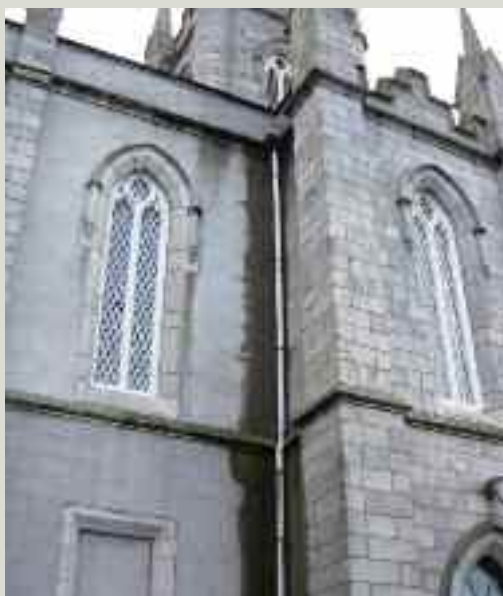
Walls will quickly become saturated if rainwater cannot be shed effectively from the roof. Staining, discolouration and plant growth behind and beside downpipes are signs of problems at eaves or parapet level that require immediate attention
