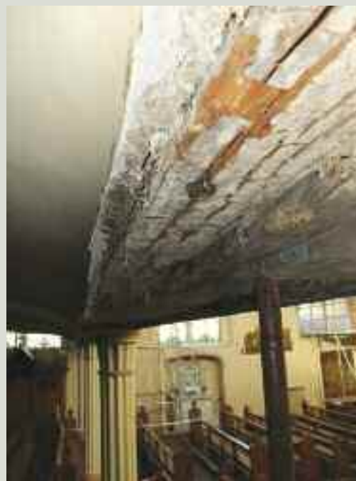
Regular inspections and scheduled maintenance work should prevent rot from taking hold to the degree that it causes structural damage, as has happened to this beam which supports an organ gallery
