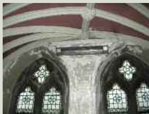
Church lighting and heating systems may evolve on an ad-hoc basis as funds become available. In this case, strip lights and electric bar heaters were fitted to some of the aisles. Conservation works to the church will include the removal of these fittings and repairs to the roof above to eradicate the damp in the wall
