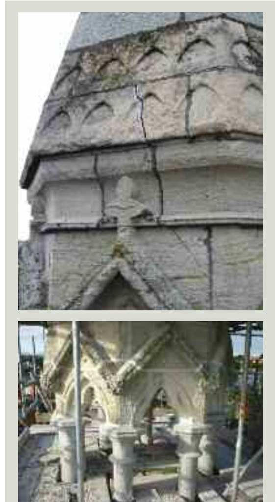
This Bath stone turret, which is also a bell-tower, is in a highly exposed location. Several stones cracked due to rusted cramps and the poor condition was exacerbated by previous misguided cementitious repair. New stainless steel collars and ties were fitted and the turret was repointed
