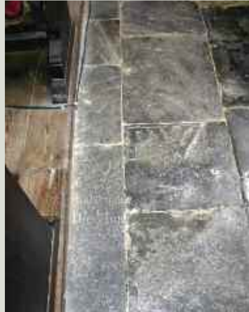
Floor surfaces may be of significance for historic or social reasons. The paving of this cathedral floor contains cut down and reused grave slabs
