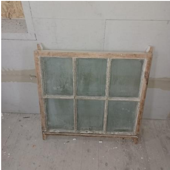
Fig.29 – Existing Window Repairs
