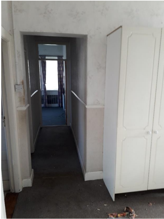
Fig.19 – Remote Hub 1 st Floor Landing 2023
