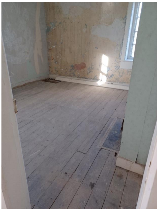
Fig.21 – Remote Hub 1 st Floor Office 2023
