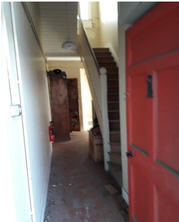
Fig.9 - Garda Station Entrance Hall 2023
