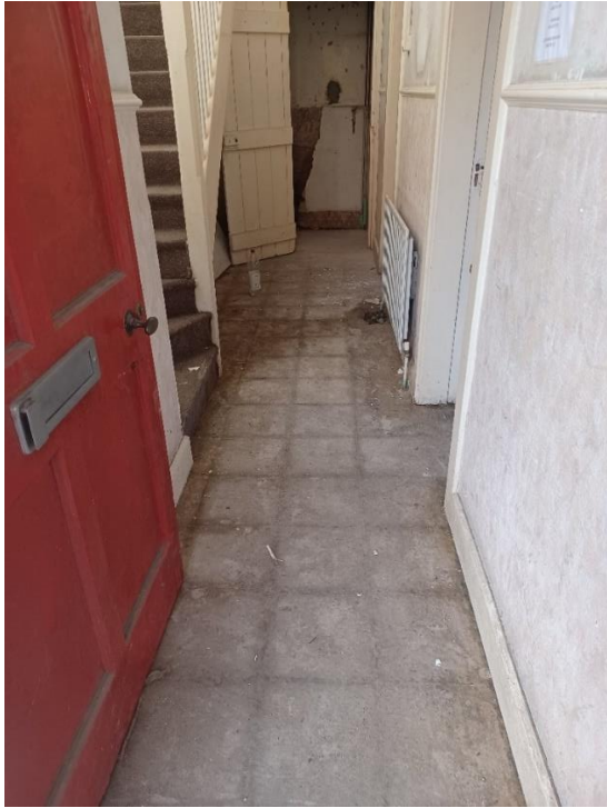
Fig.23 – Remote Hub Entrance Hall 2023
