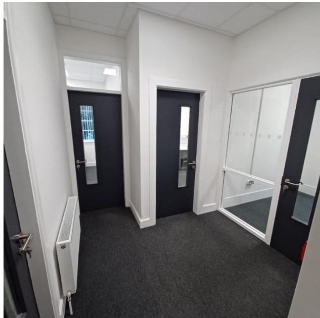
Fig.20 – Remote Hub 1st Floor Landing 2024
