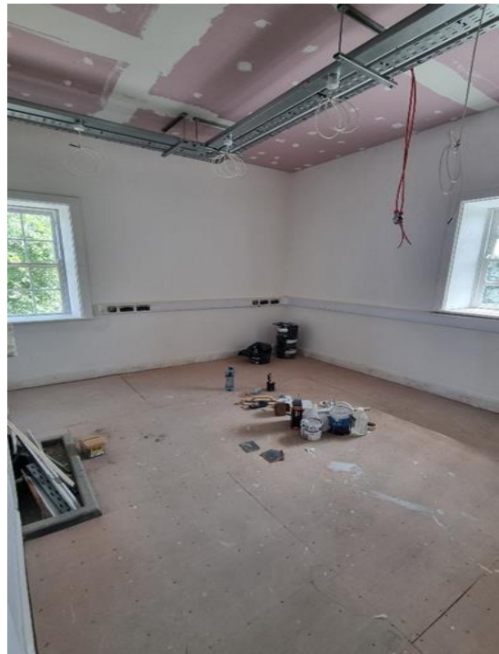
Fig.30 – First floor overlay -fire upgrade
