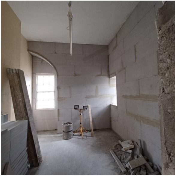
Fig.7 – Garda Station Back Office 2024 – Calsitherm Insulation
