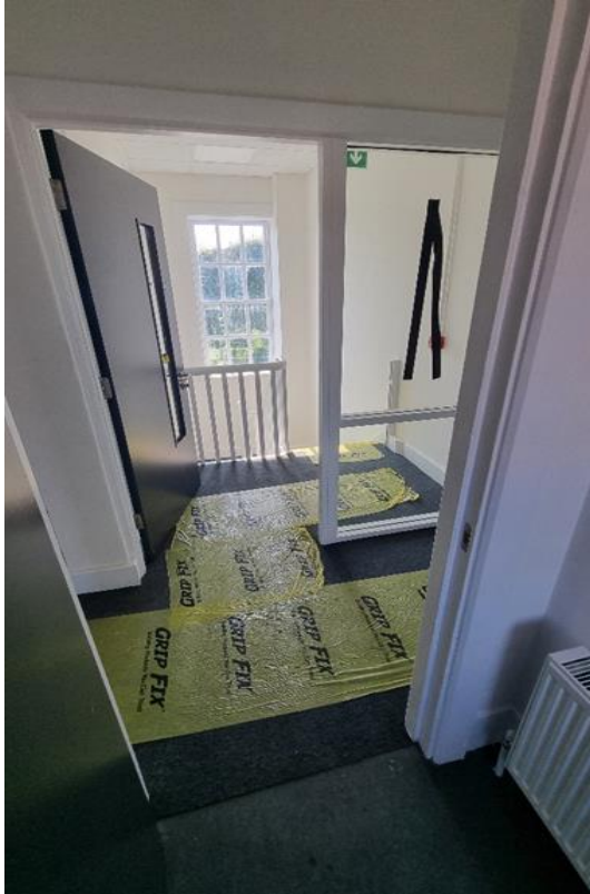
Fig.31 – Fire door and screen to stair enclosure
