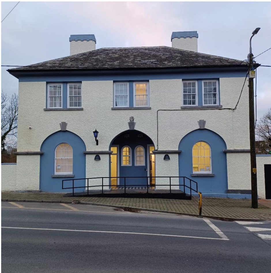
Fig.2 – Front Elevation 2024 – Existing colour scheme maintained
