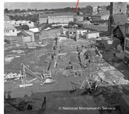
Phase 2 Monitoring, looking north
