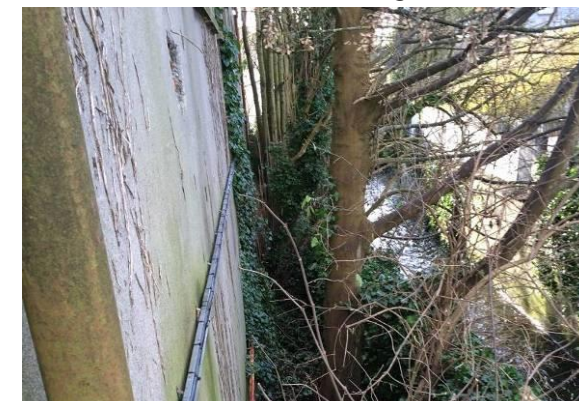
View west long walkway between Mayfair and Breaghagh River
