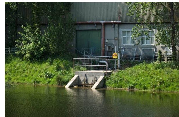
View west from John's Quay of West Bank and drainage outfall
