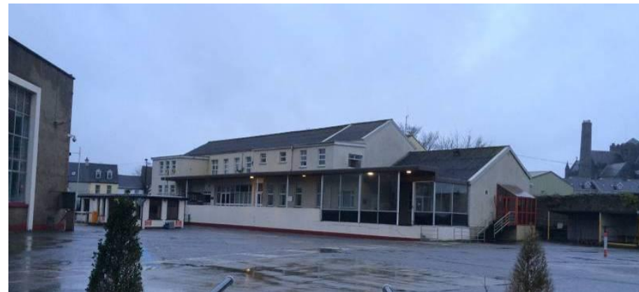
View from St. Francis Abbey west to Mayfair Building
