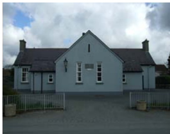
The Old School House now in use as a Community Centre
