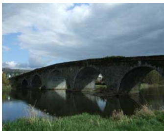
Protected Structure: Bridge over River Nore
