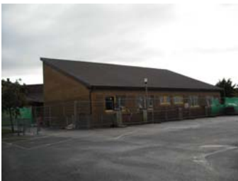
Recently Completed Extension to Primary School
