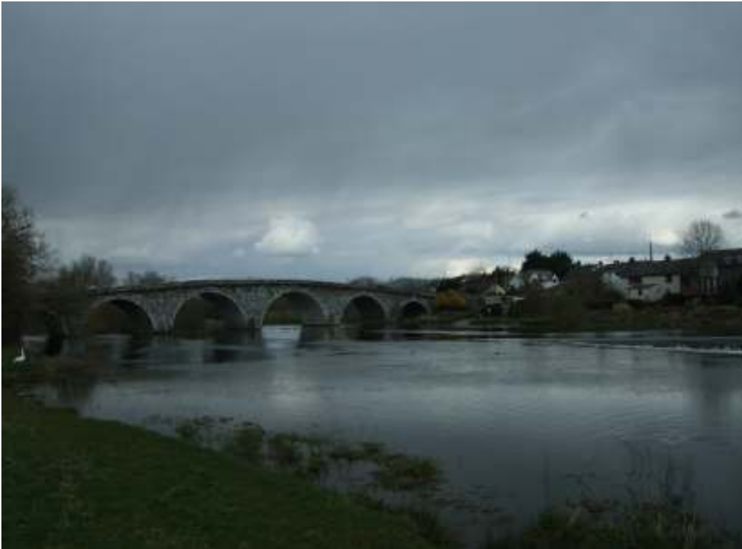
Figure 4: Looking northeast across river towards the bridge
