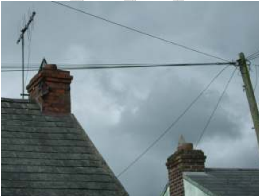
Figure 10: Gable ended chimneystacks
