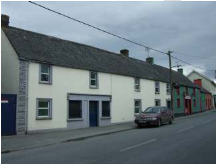
Figure 2: Terraced structures along Main Street
