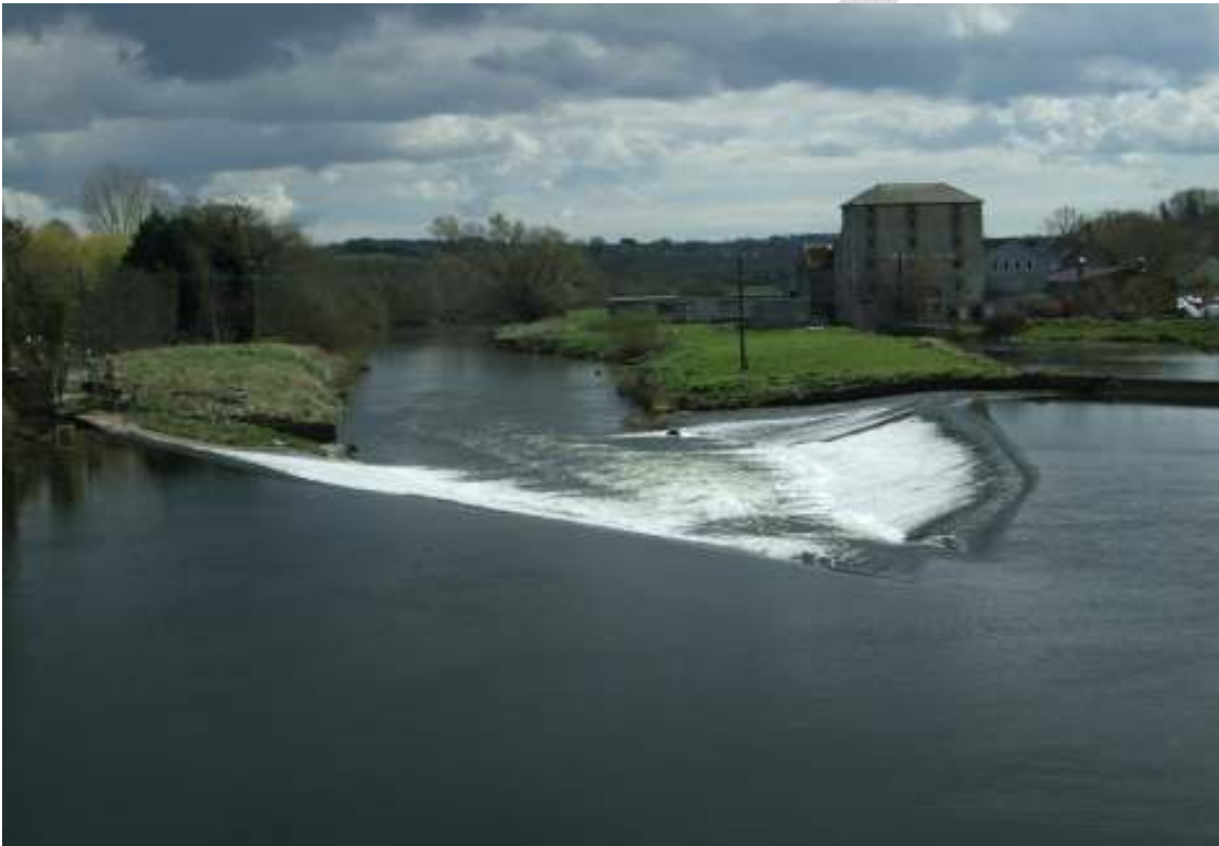
Figure 3: Mosse mill with weir to foreground
