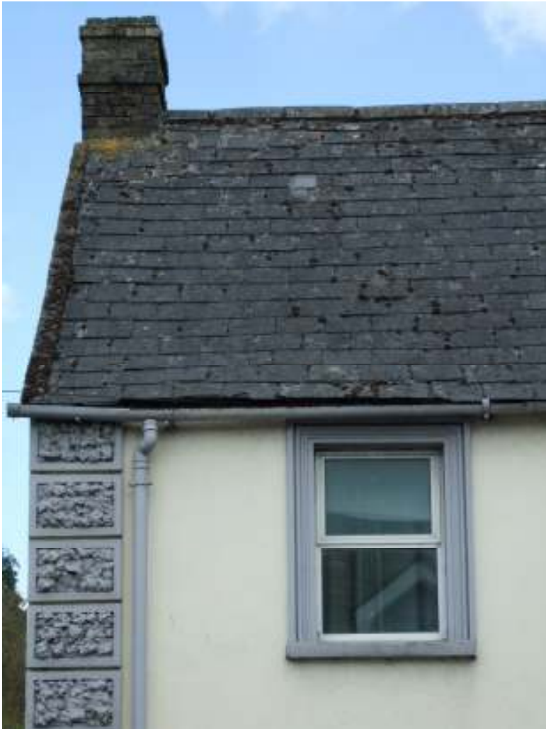
Figure 11: Slate, stone and timber, render and decorative render mouldings used in the finish of buildings
