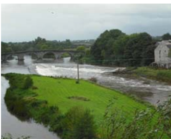
View northwards of Bridge, Weir and Kells Mill
