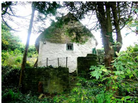
Side of cottage
