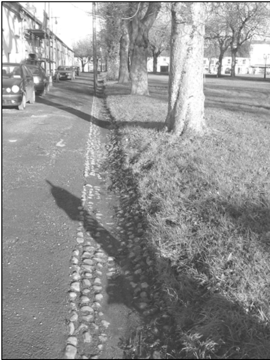
Cobbled open gutter at New Row
