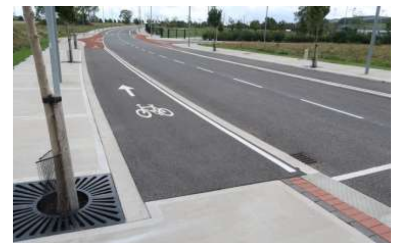
Figure 4.54: Extract from page 86 of the National Cycle Manual illustrating how to re-establish from an Off Road Cycle Track to Cycle Lane on approach to a junction. This design can be adapted to cater for on-street parking by placing spaces within the green area or verge between the vehicular carriageway and Cycle track.
