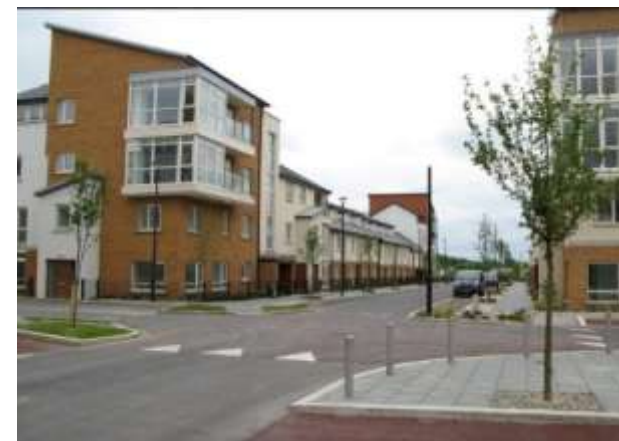
Figure 4.53: Example of a narrow verge between a cycle track and on-street parking. This verge provides a buffer that protects cyclists from opening doors.
