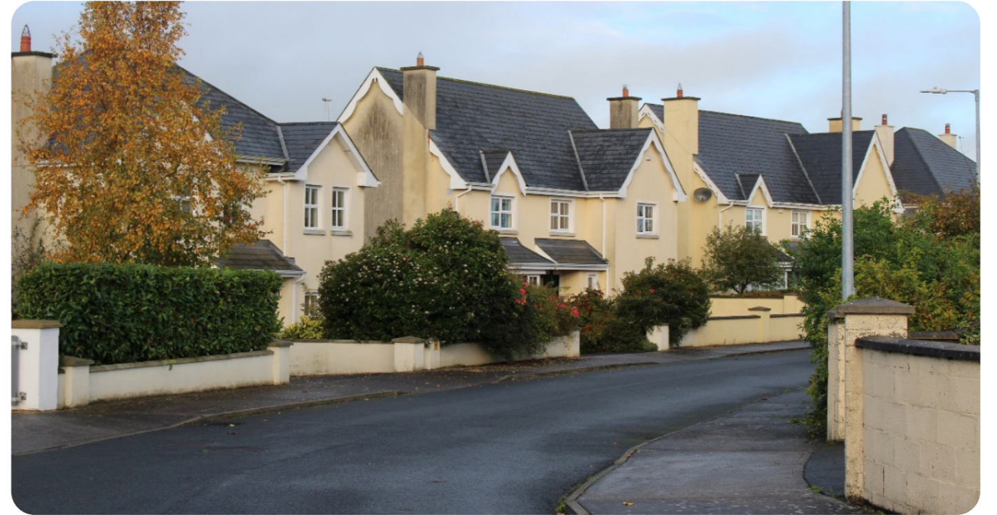
Figure 3.11: Housing Stock in Ballyragget (address: Bridge Street).
