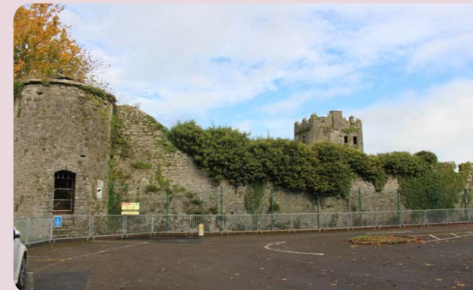
Ballyragget Castle and Castle Walls
