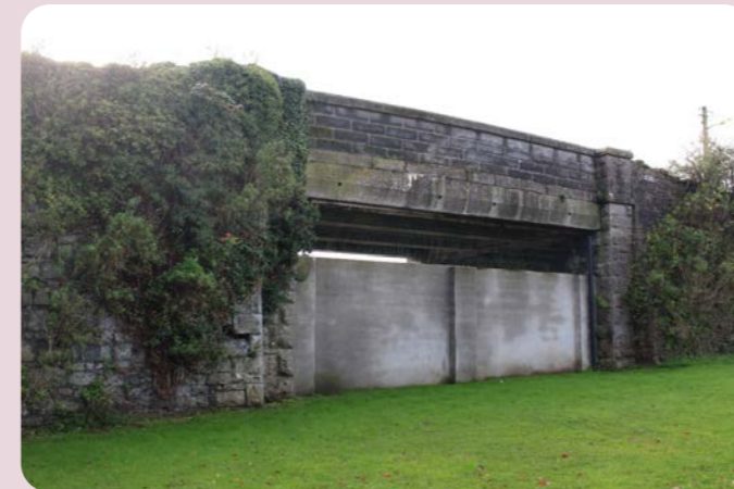
Old Railway Bridge
