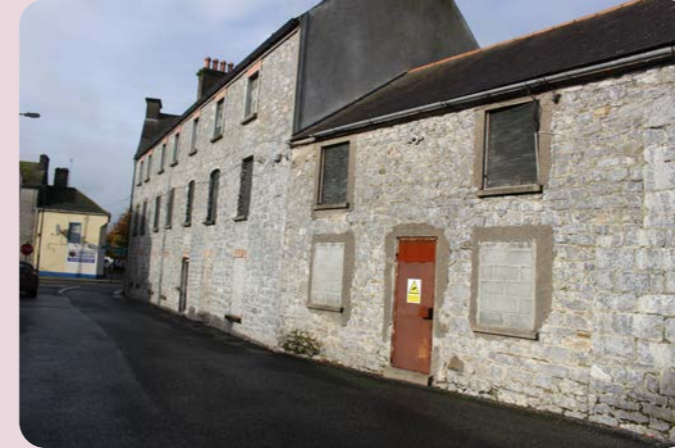
Butler's House from the rear
