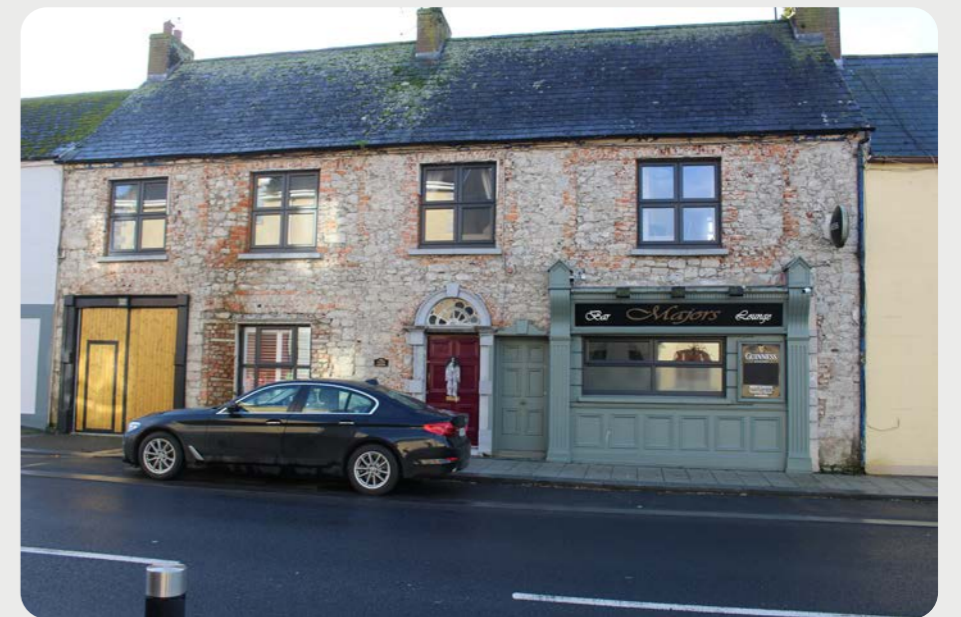
Figure 3.29: House on the Square (NIAH Ref. 12303005)
