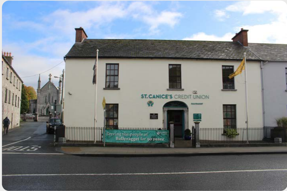
Figure 3.33: St. Canice's Credit Union, Ballyragget.
