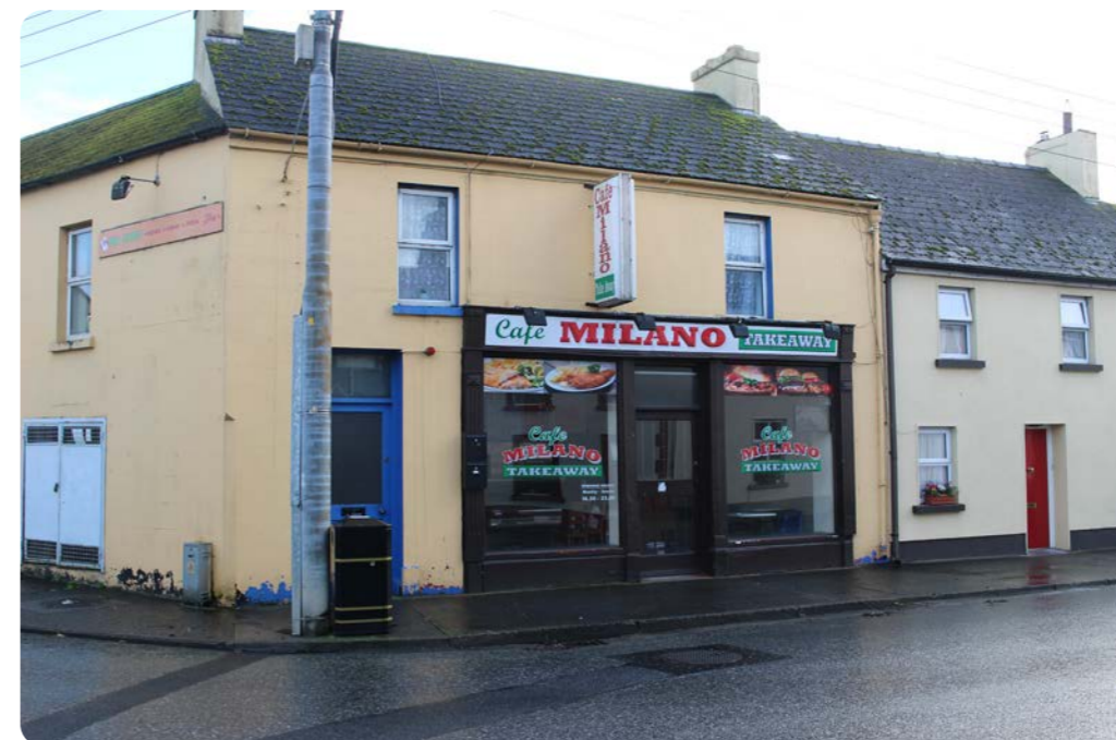
Shopfront Clutter in Architectural Conservation Area
