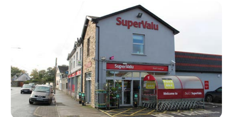
Figure 3.31: Supervalu Supermarket in Ballyragget
