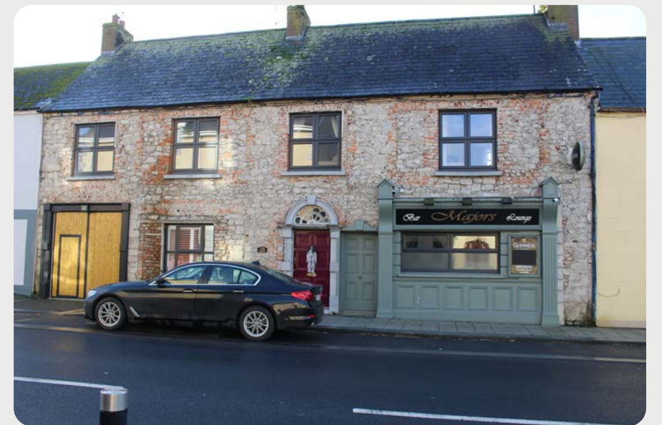
Figure 3.29: House on the Square (NIAH Ref. 12303005)
