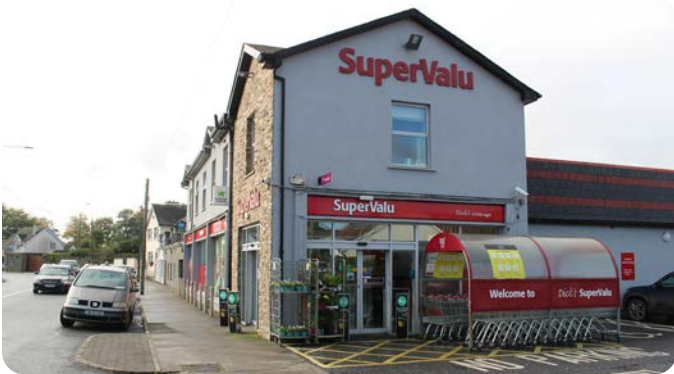
Figure 3.31: Supervalu Supermarket in Ballyragget
