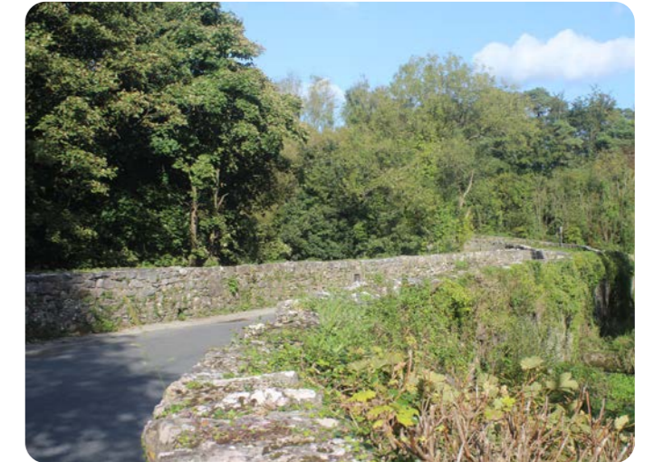
Figure 2.4: Kilmacow Bridge, Lower Kilmacow
