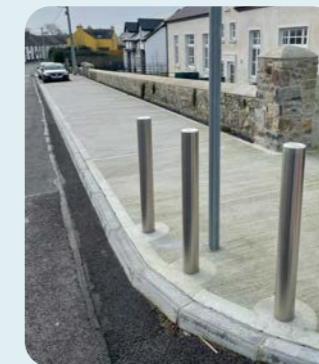
Figure 3.35: Improved footpaths at the Old Creamery
