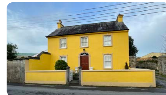
Figure 5.21: Former Greenvale Mill
