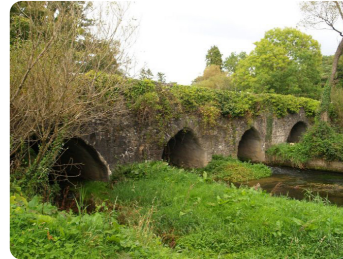
Figure 2.3: Kilmacow Bridge at River Blackwater (Source: Kilkenny County Council)
