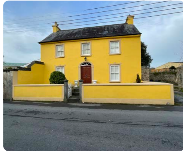
Figure 3.24: Protected Structure - Narabane South
