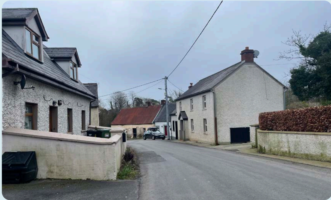
Figure 3.13: Absence of footpaths, Kilmacow lower
