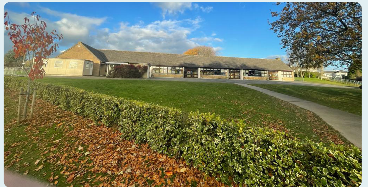
Figure 3.23: St Senans National School Senior Building
