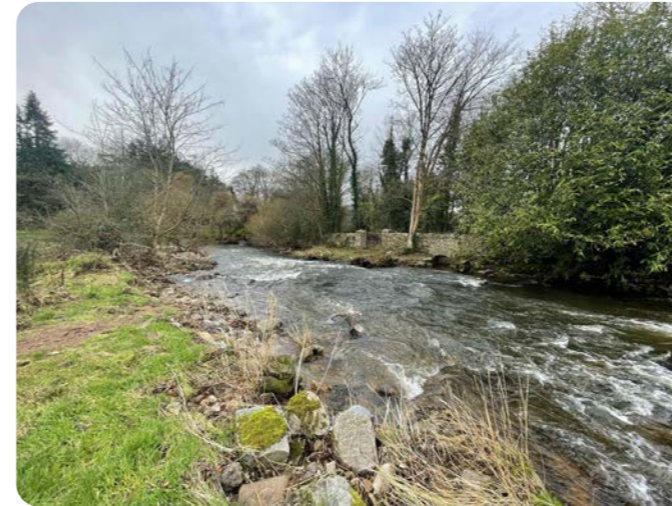
Figure 2.9: View of the River Blackwater from below the weir
