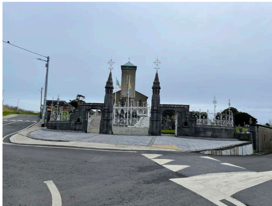
Figure 5.30: Protected Structure: Saint Senans Church
