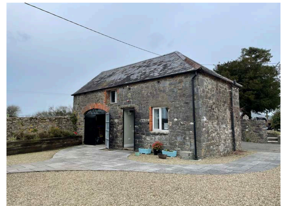
Figure 5.31: Protected Structure: The cottage in Narabane
