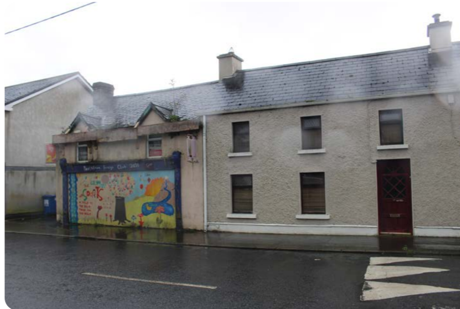
Figure 5.14: Derelict building on Main Street.
