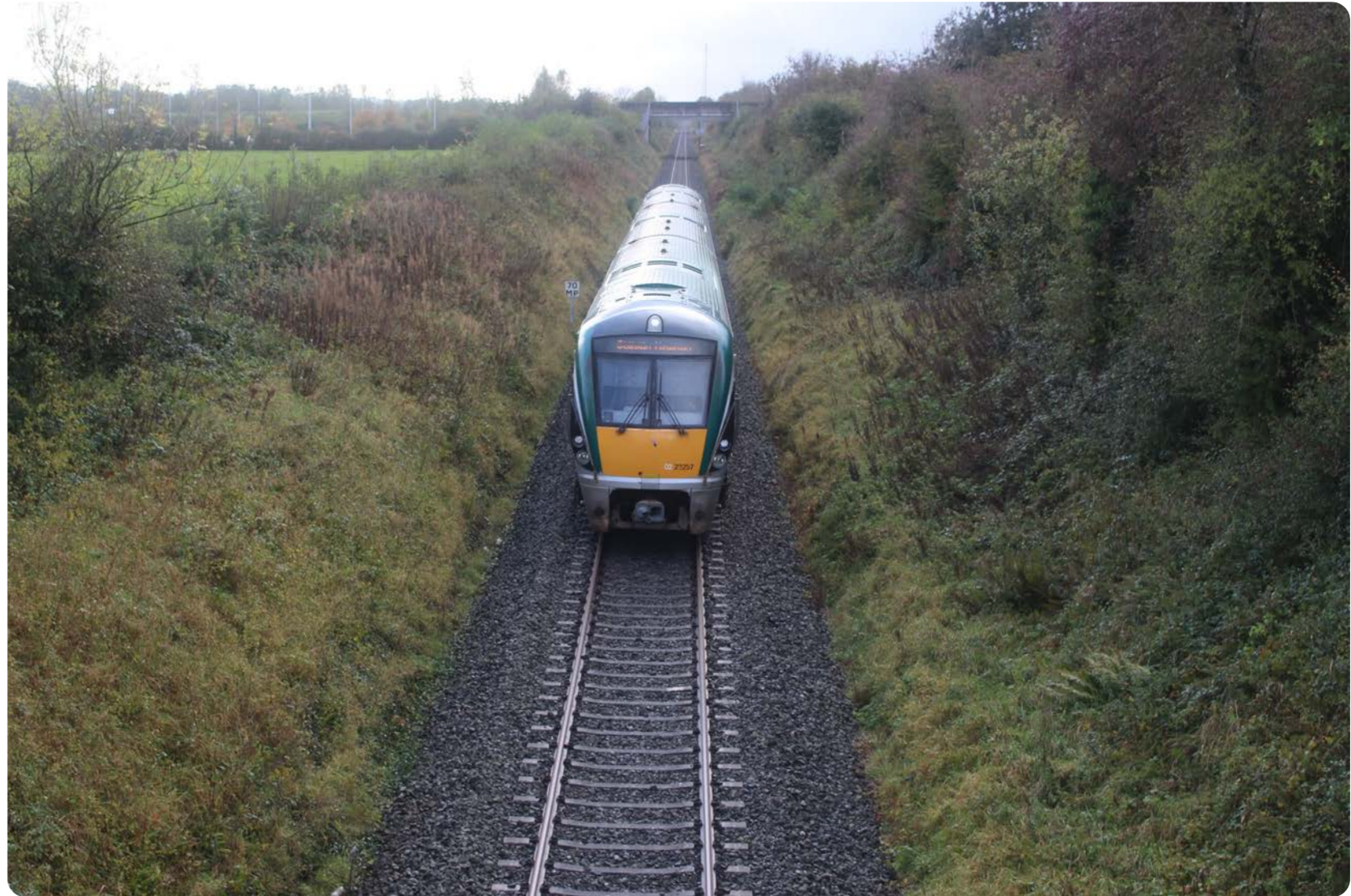
Figure 5.13: Railway along the western boundary of Paulstown.
