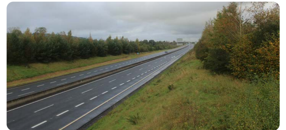
Figure 3.26: The M9 Motorway from the An Choill Rua Bridge
