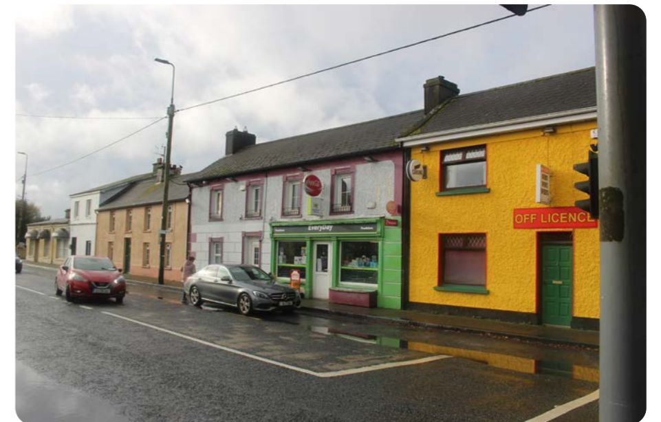
Figure 5.17: Facades along R712
