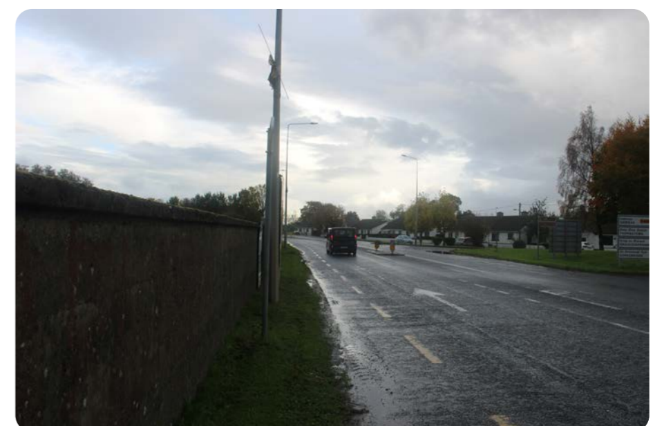
Figure 5.9: No Footpath along the R448
