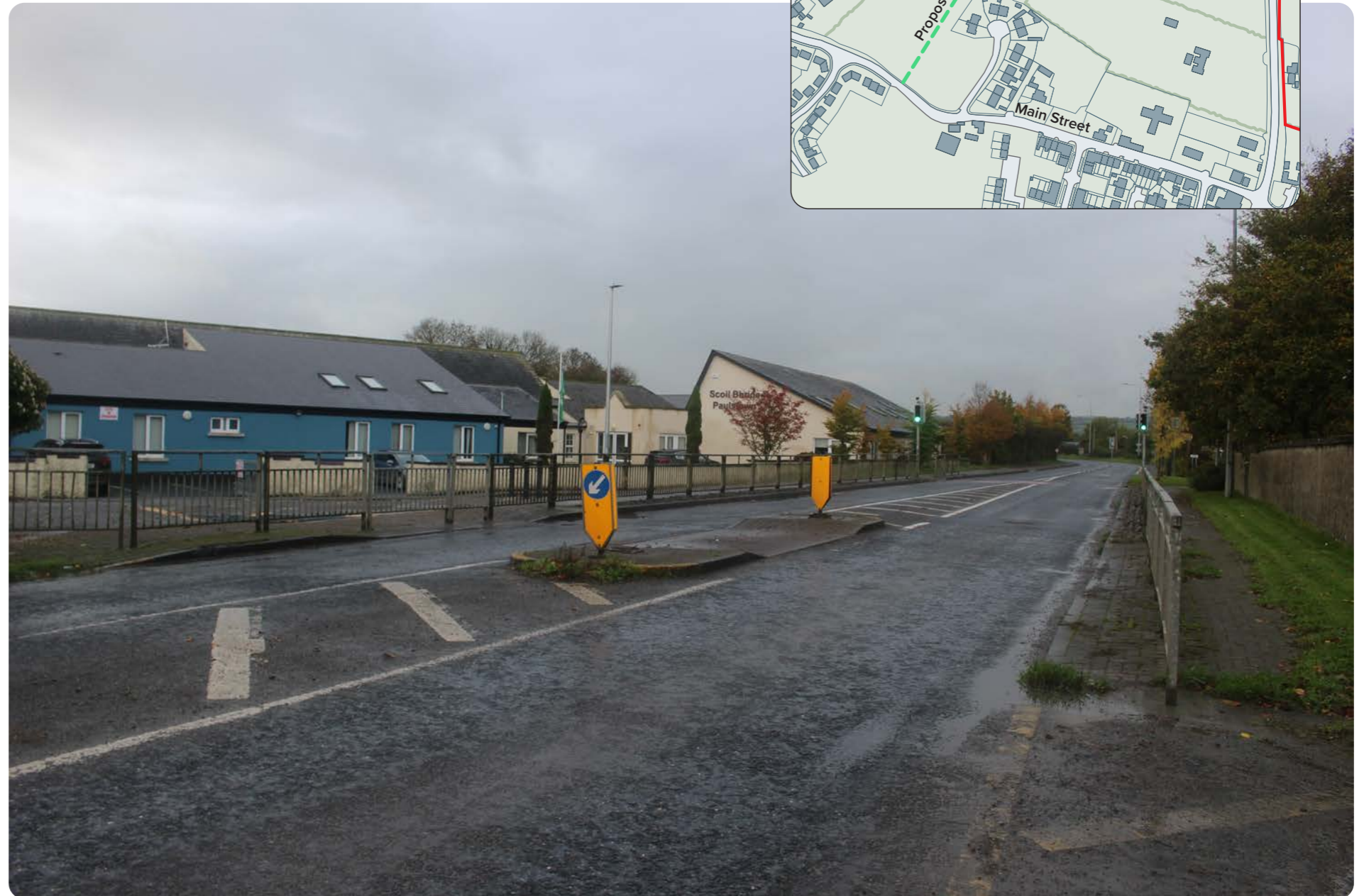
Figure 5.3: Scoil Bhride walkway
