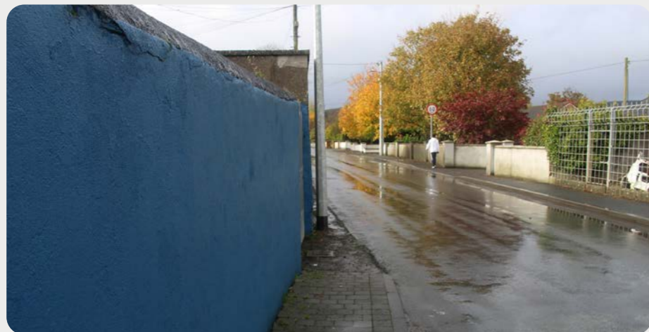
Figure 3.33: Pavement disappears along An Choill Rua
