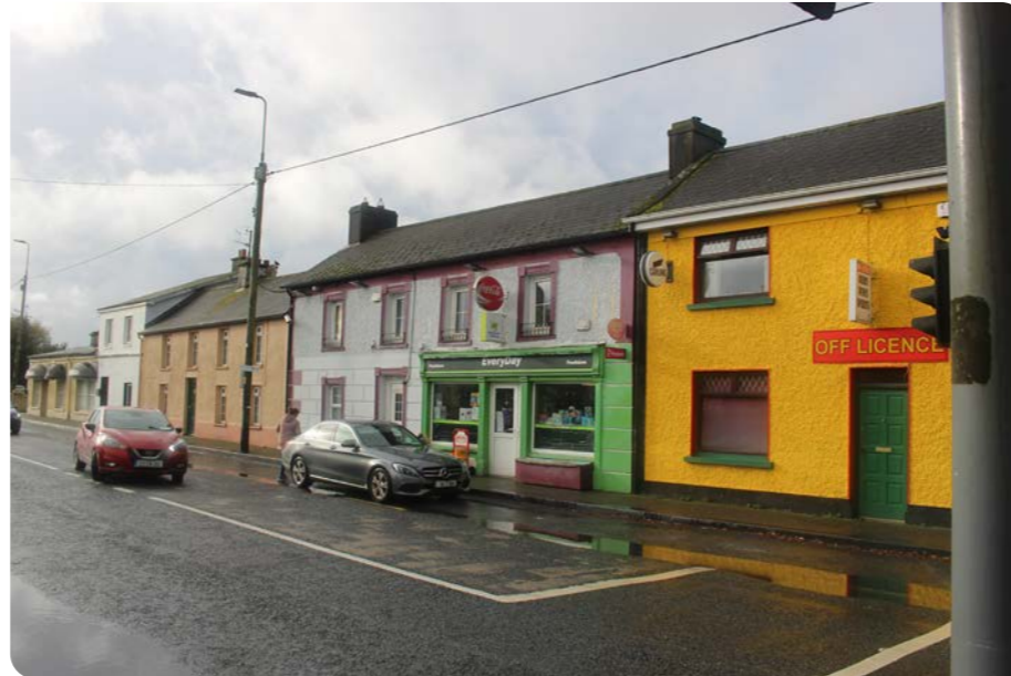
Figure 5.6: Narrow Footpaths along the R712.
