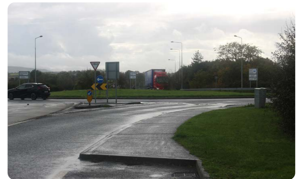
Figure 5.2: Roundabout approaching Paulstown from the M9 Motorway.
