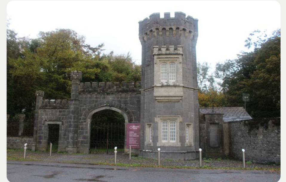
Figure 3.14: Shankill Castle and Gardens southern entrance.
