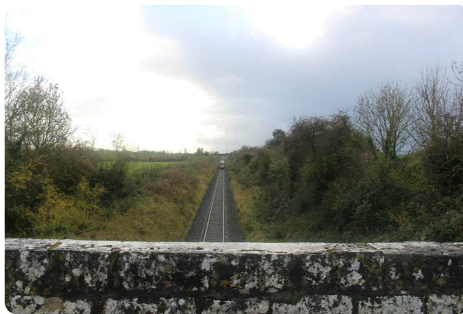
Figure 3.29: Dublin-Waterford Railway line running along the western boundary of Paulstown
