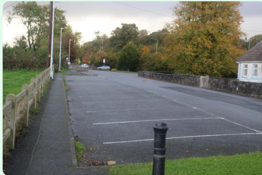
Figure 5.4: Carpark at Paulstown Health Centre - Landscaping Intervention
