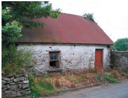
Traditional vernacular single storey cottage with corrugated iron roof
