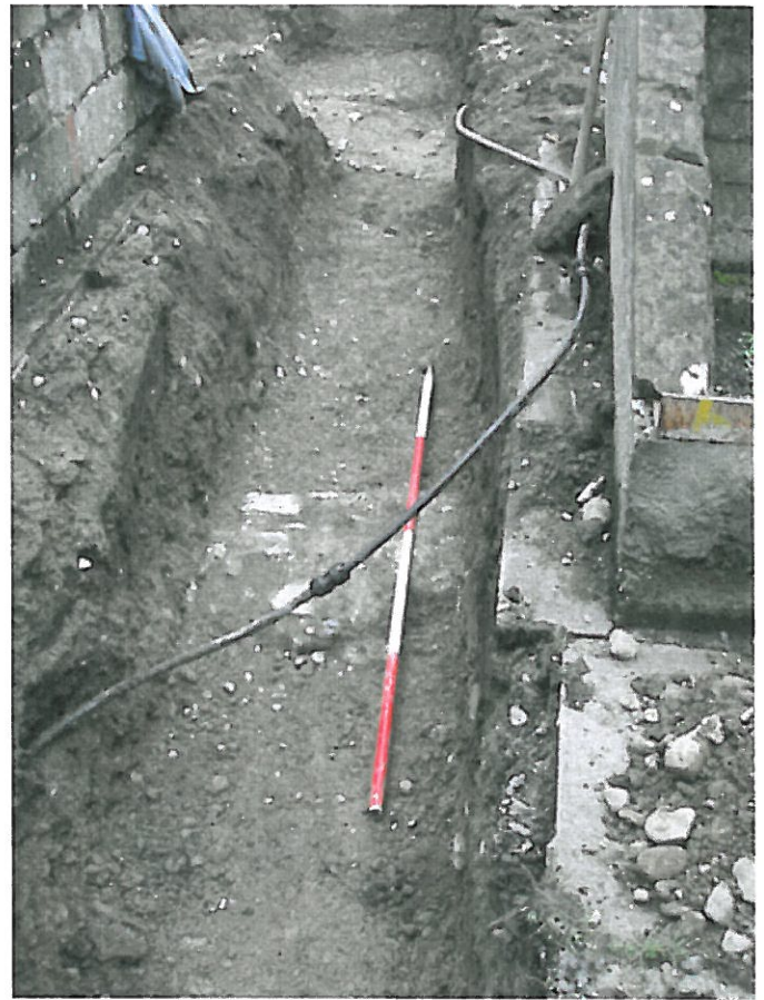
Plate 2. Wall footing F1 in trench 1A, looking north.
