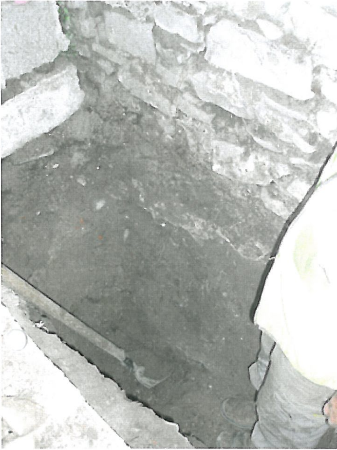
Plate 11. Trial pit 1, shovel at base of wall.
