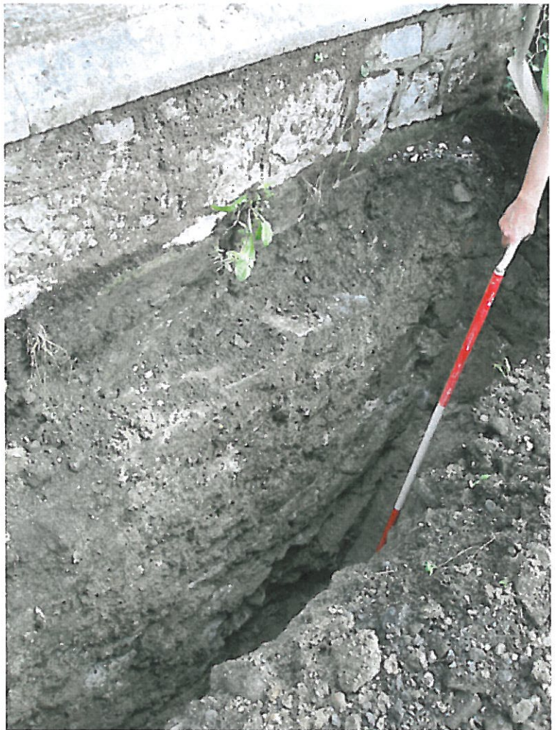
Plate 17. Trial pit 7, wall of Evans Home on plinth footing.
