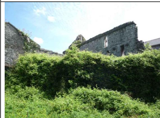
Fig.41: Blanket vegetation to the outdoor sanitary block to the southeast of site.
