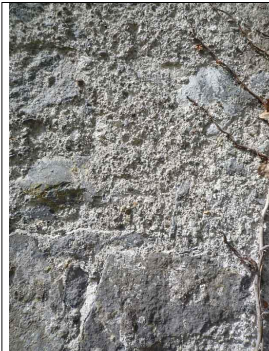
Fig.27: Area of surviving harling to the west elevation of the main block.
