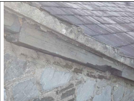
Fig.20: Detachment of stonework from the raking stringcourse to the pedimented breakfront to the main block.
