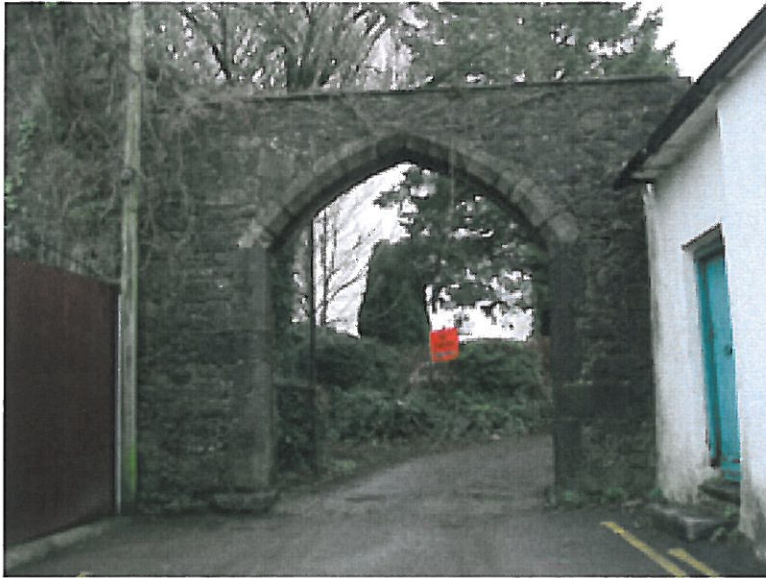
Plate 39. Gate arch at Barrack Lane, three phases of construction evident.
