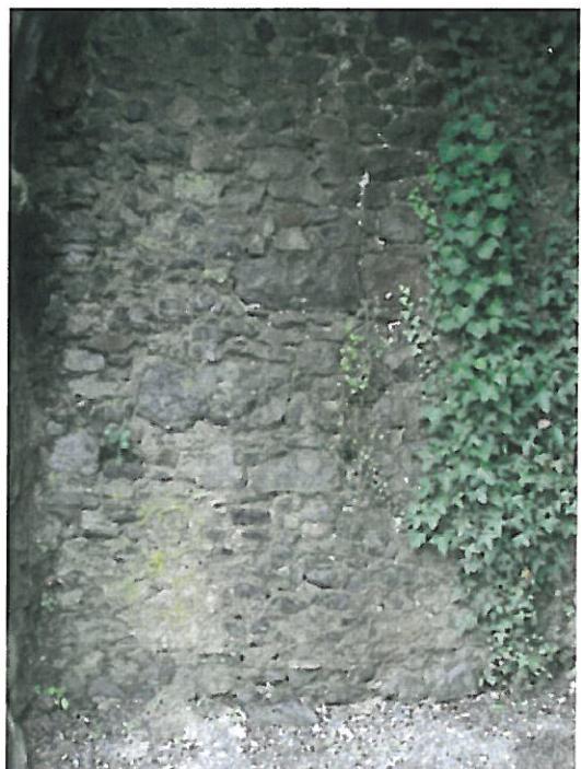
Plate 28. Detail of masonry, int north wall.
