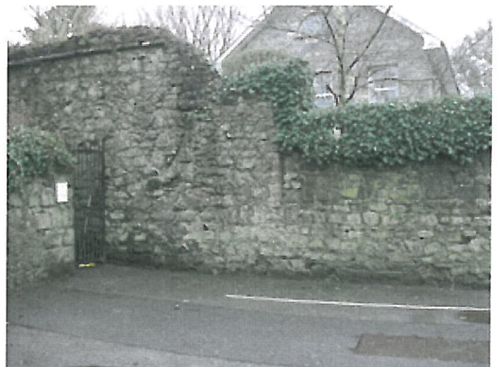
Plate 22. North wall claustral building, with added masonry to west, with brick dressed window.
