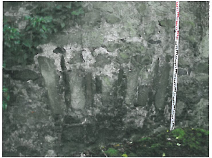
Plate 35. Voussoirs of arch over blocked ope 4.
