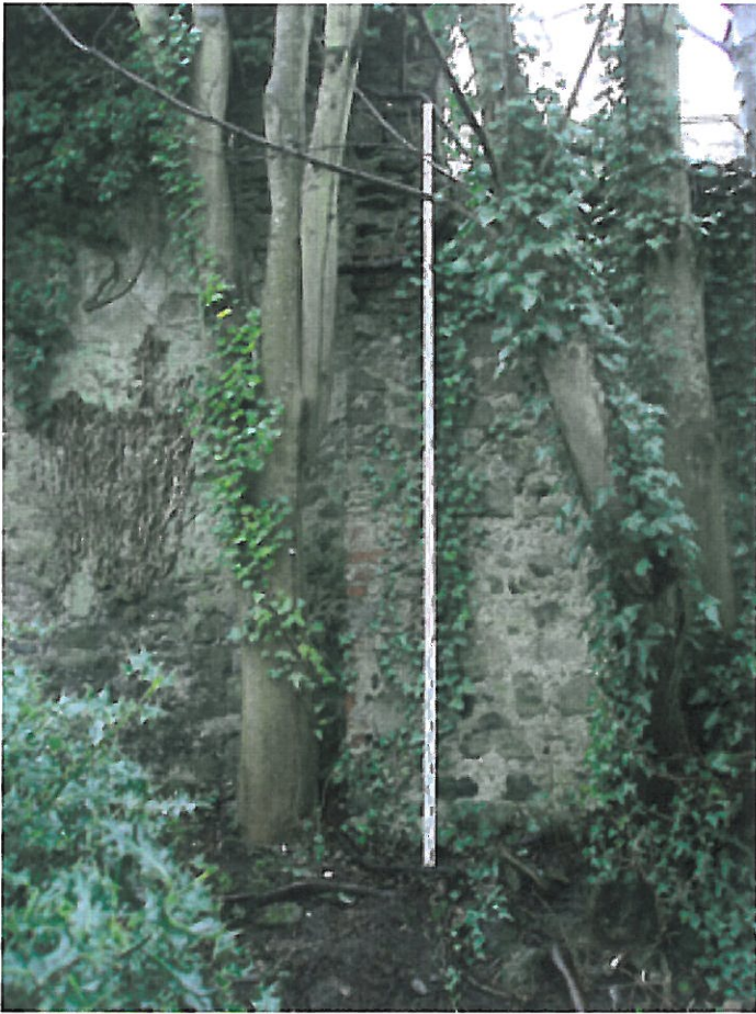
Plate 34. Brick trimmed projection where walls of two buildings on Rocque meet.
