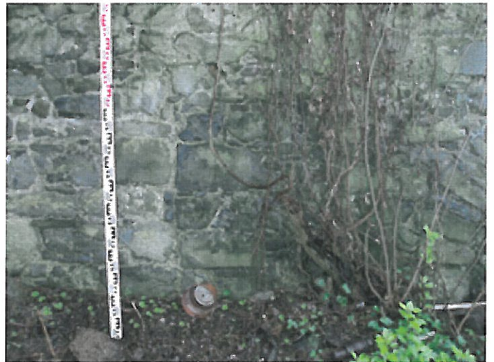
Plate 32. Join/ abutment of walls, west boundary wall.
