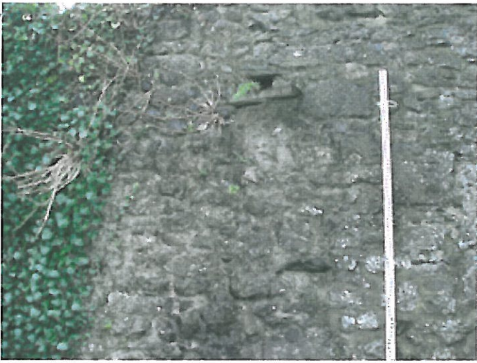
Plate 23. Drip spout in north wall, claustral building.
