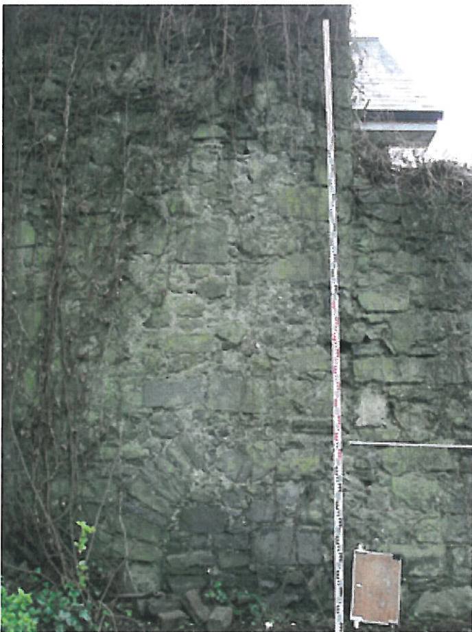
Plate 31. Blocked arch, cut /abuted by later wall.
