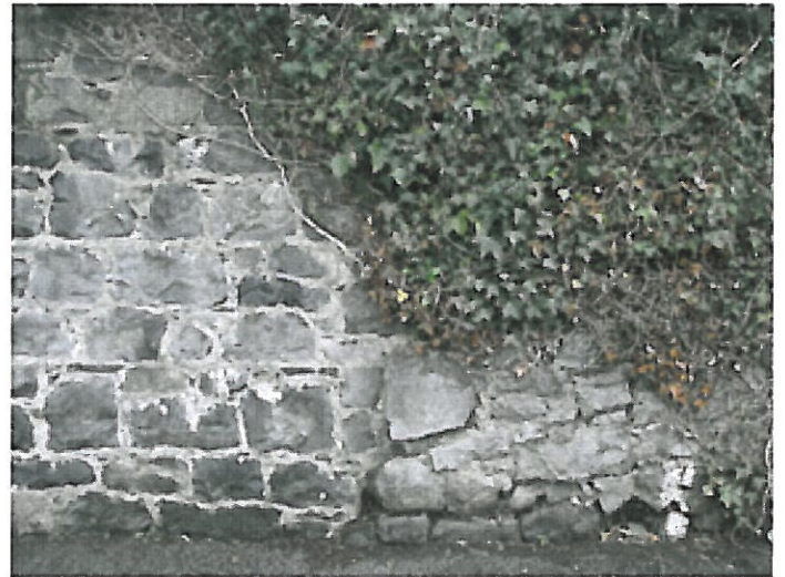
Plate 18. Wall along millrace, showing join of two builds.
