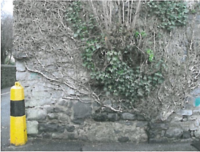
Plate 17. Wall along millrace with flat headed blocked ope.
