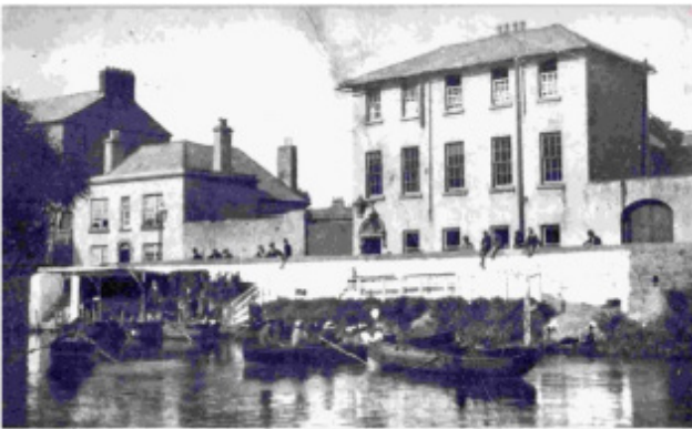
Figure 5-7. Historical photograph of John's Quay South. Source: Kilkenny Co.Co.
