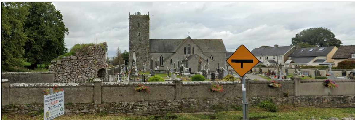
Plate A10.1 General View of CH-1 from south
