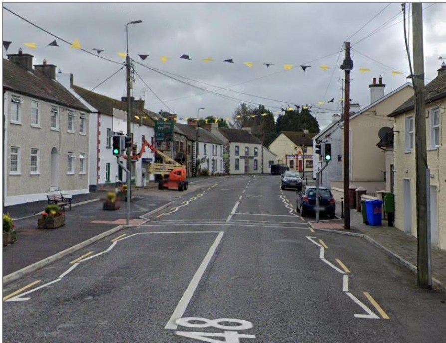
Figure 15-6 - Signalized Pedestrian Crossing in R448
