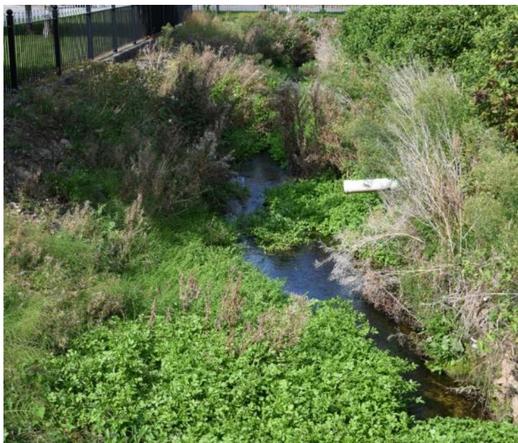
Plate 5. Section D showing discharge pipe from bank.
