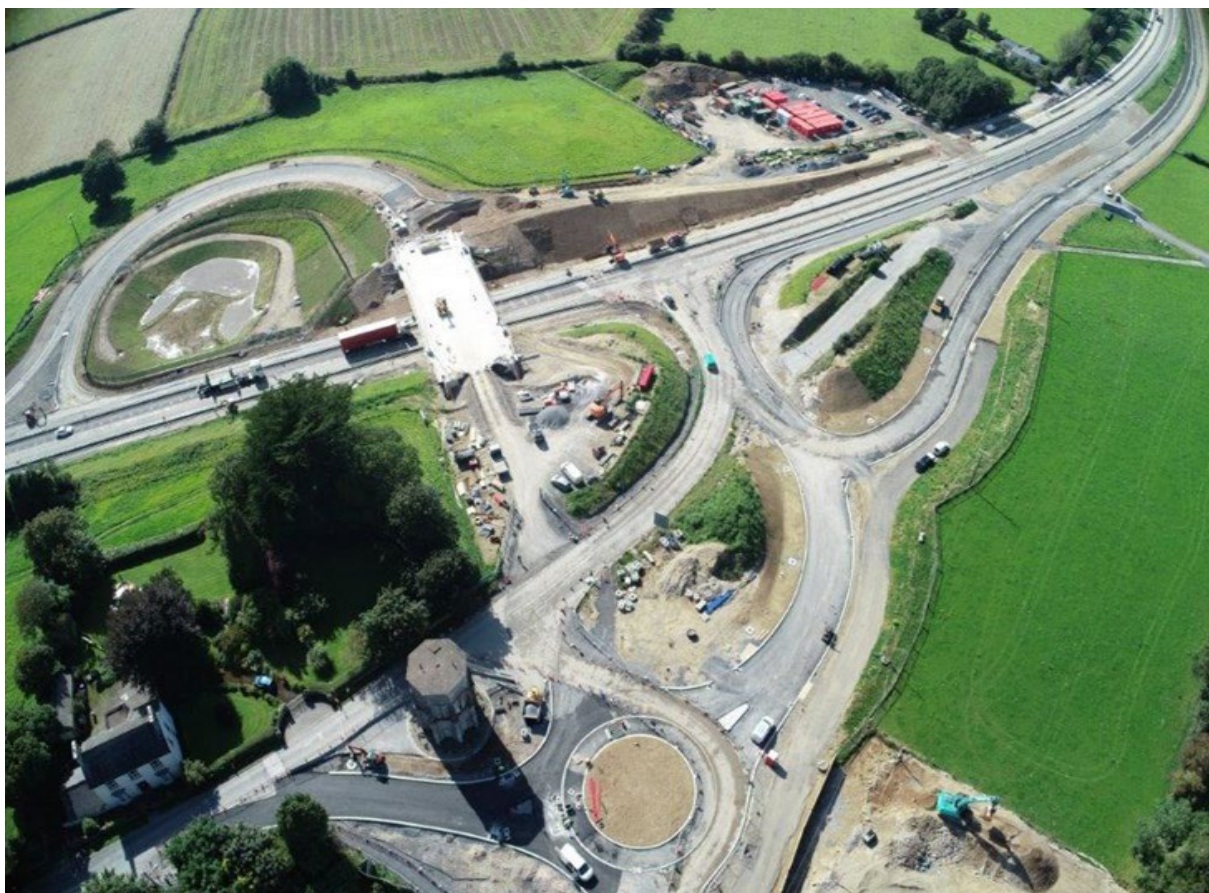
Overhead View of the Tower Road Project
