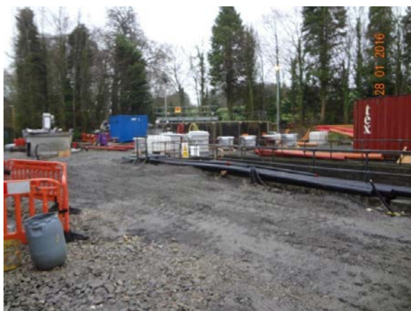
Castlecomer Wastewater Treatment Plant - Works in Progress
