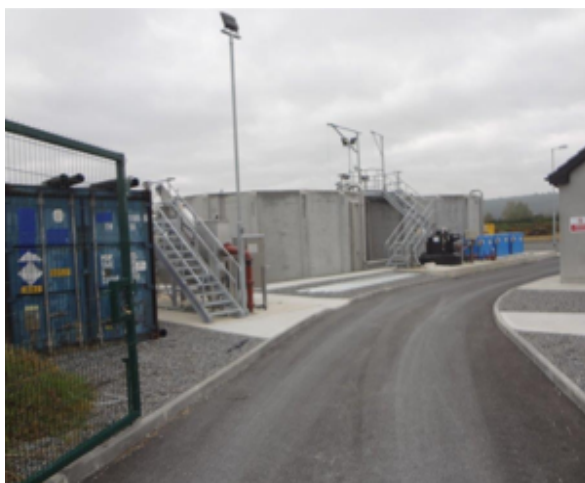
Freshford Waste Water Treatment Plant
