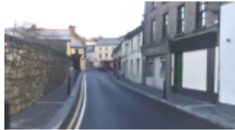
Pipe Street – After
