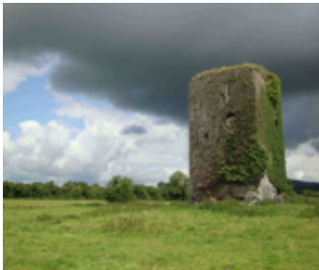
Castle Field, Sandfordscourt
