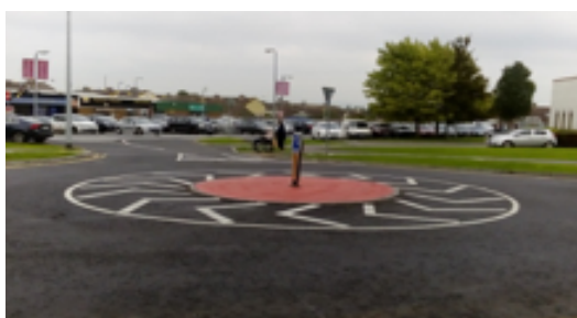
Completed works at Bohernatounish Road
