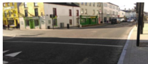
Irishtown Junction Before Works
