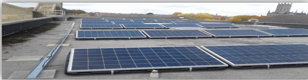
Kilkenny Fire Station 6kWp solar photovoltaic panels
