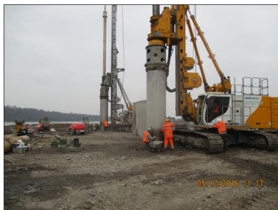
Piling Works at Pier 3 at Pink Rock.
