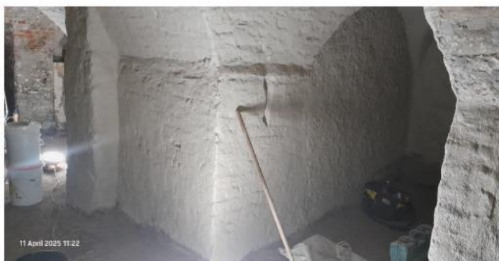
Limewash ongoing in basement
