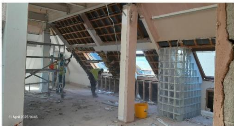
Removing plaster slab and fibreglass insulation on fourth floor
