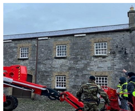
Swift Nest Boxes installation in progress at James Stephens Army Barracks
